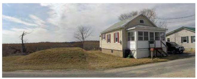
**Figure 12.9** Mounds-based septic system next to house along the back side of Pickering Beach, Delaware (March 2009). [Photo source: <sup>©</sup>James G. Titus, used with permission].
