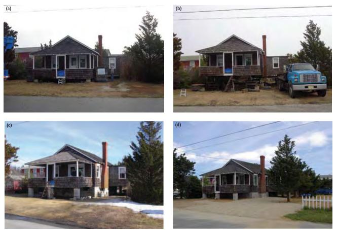
**Figure 12.5** Elevating land and house (January through June 2005). (a) Initial elevation of house in Brant Beach, New Jersey. (b) Structural beams placed under house, which is lifted approximately 1.5 meters by hydraulic jack in blue truck. (c) Three course of cinder blocks added then house set down onto the blocks. (d) Soil and gravel brought in to elevate land surface. [Photo source: <sup>©</sup>James G. Titus, used with permission].
