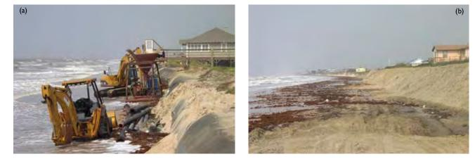
Figure 6.2 Geotube (a) before and (b) after being buried by beach sand at Bolivar Peninsula, Texas (May 2003) [Photo source: <sup>®</sup>James G. Titus, used with permission].
