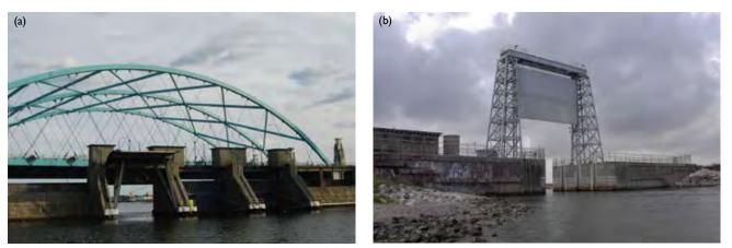
**Figure 6.6** Storm surge barriers. (a) Fox Point Hurricane Barrier and Providence River Bridge, Providence, Rhode Island (August 2008) and (b) Moses Lake Floodgate, Texas City, Texas (March 2006) [Photo sources: (a) Marcbela; (b) <sup>©</sup>James G. Titus, used with permission].
