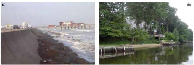
**Figure 6.1** Seawalls and bulkheads (a) Galveston Seawall in Texas (May 2003) and (b) bulkheads with intervening beach along Magothy River in Anne Arundel County, Maryland (August 2005) [Photo source: <sup>©</sup>James G. Titus, used with permission].
