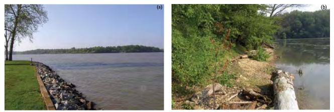
**Figure 12.4** Hard and soft shore protection. (a) Stone revetment along Elk River at Port Herman, Maryland (May 2005). (b) Dynamic revetment along Swan Creek, at Fort Washington, Maryland (September 2008) [Photo source: <sup>©</sup>James G. Titus, used with permission].
