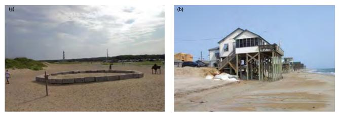
**Figure 6.8** Relocating structures along the Outer Banks (a) Cape Hatteras Lighthouse after relocation at the Cape Hatteras National Seashore, Buxton, North Carolina (June 2002); the original location is outlined in the foreground, and (b) a home threatened by shore erosion in Kitty Hawk, North Carolina (June 2002) The geotextile sand bags are used to protect the septic system [Photo source: <sup>©</sup>]ames G. Titus, used with permission].
