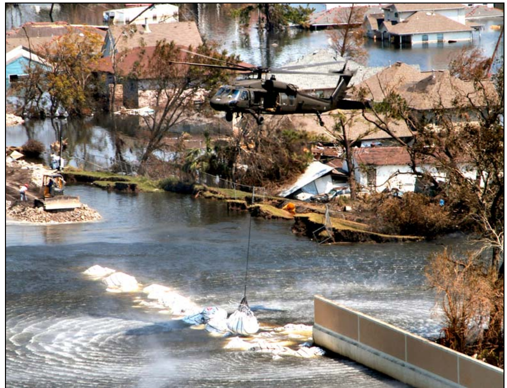
Levee Breach at the 17 th Street Canal in New Orleans, LA – Photo: US Army Corps of Engineers (2005)
