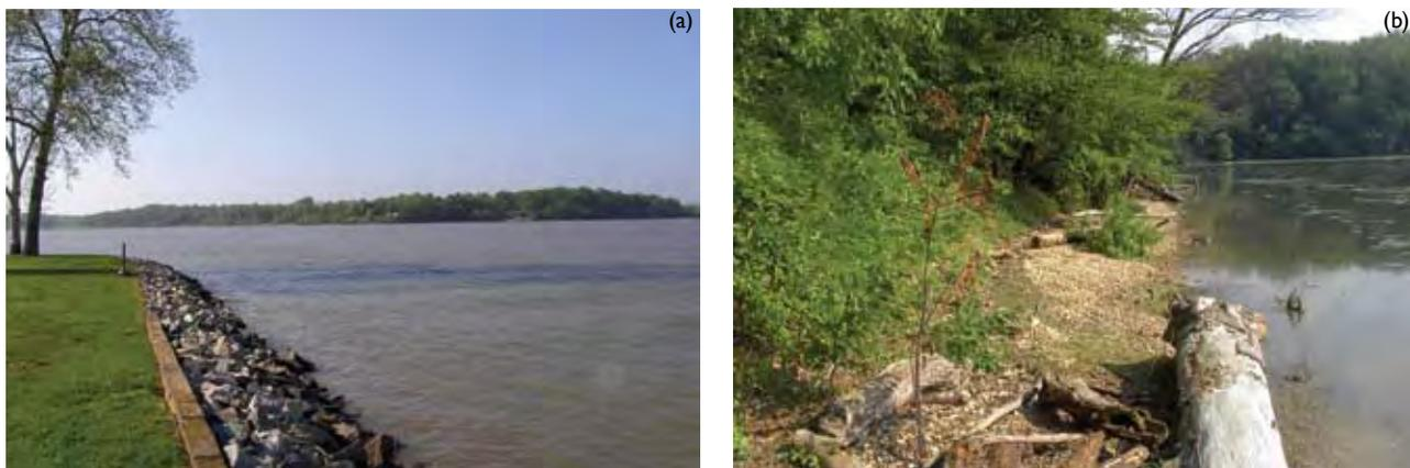
**Figure 12.4** Hard and soft shore protection. (a) Stone revetment along Elk River at Port Herman, Maryland (May 2005). (b) Dynamic revetment along Swan Creek, at Fort Washington, Maryland (September 2008) [Photo source: ©James G. Titus, used with permission].
