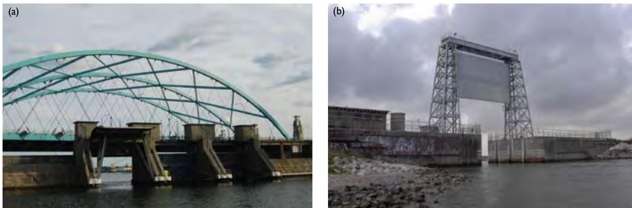
**Figure 6.6** Storm surge barriers. (a) Fox Point Hurricane Barrier and Providence River Bridge, Providence, Rhode Island (August 2008) and (b) Moses Lake Floodgate, Texas City, Texas (March 2006) [Photo sources: (a) Marcabela; (b) ©James G. Titus, used with permission].
