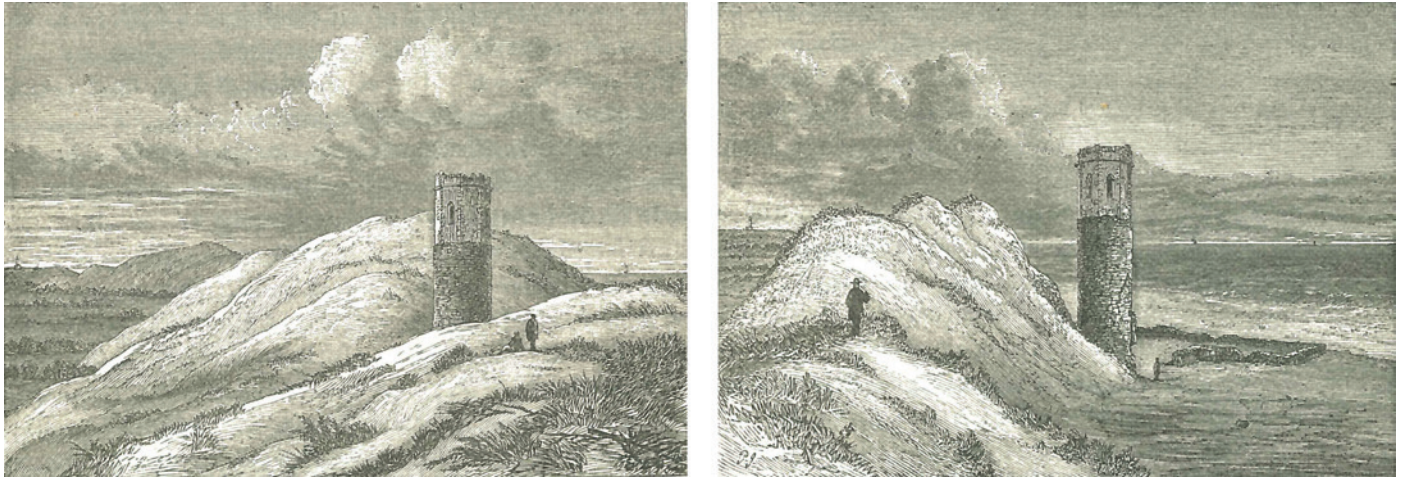
Figure 2 | Tower of the buried church of Eccles, from Charles Lyell's Principles of Geology 12 , illustrating the 'waste of the coast of Norfolk'. Left; the tower in 1839, showing the inland slope of the hills of blown sand. Right, a view of the tower from nearly the same position, as it appeared after the storm of November 1862, showing waves reaching the foundations.
