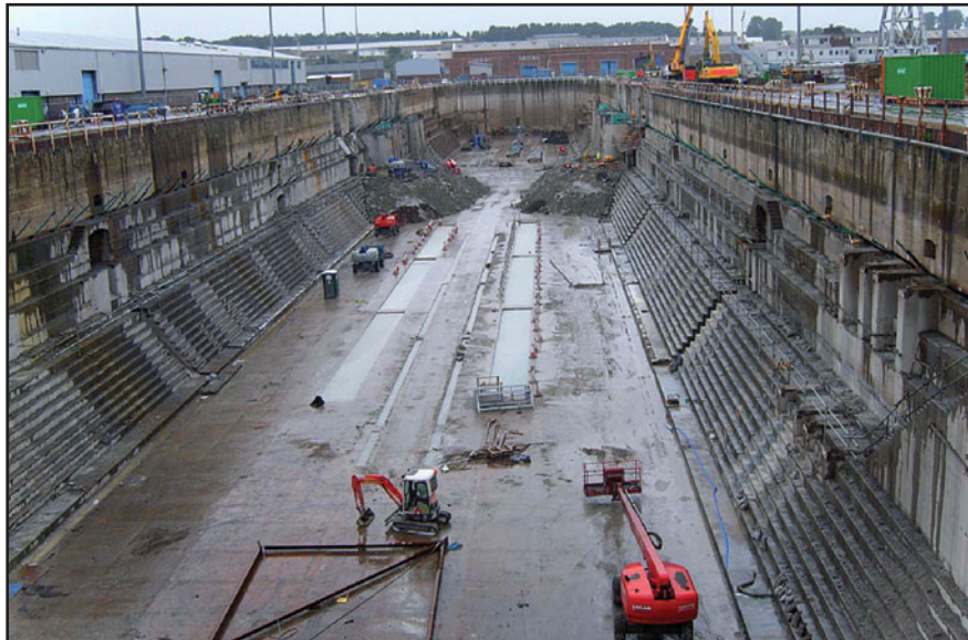
Figure F.4 Widening Work on Rosyth Dock 1
