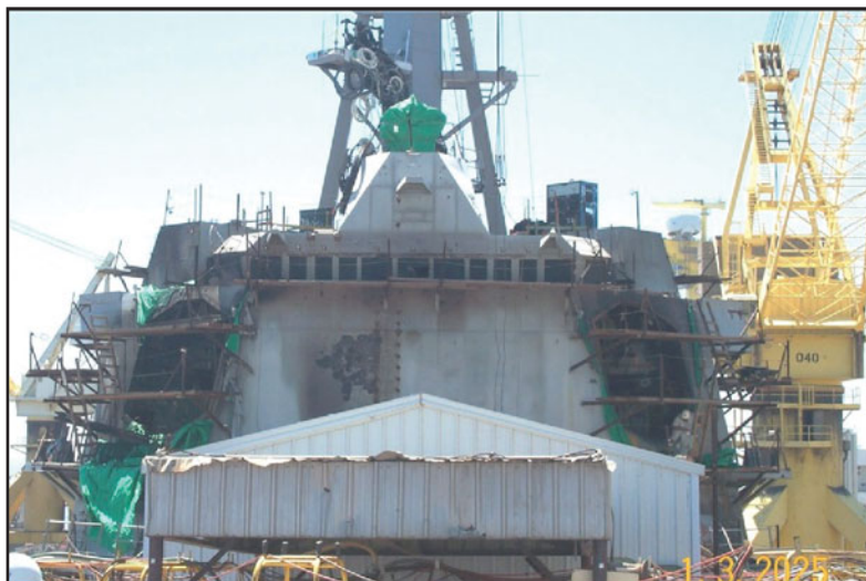
Figure A.1 View of the DDG-103 Deckhouse After an Electrical Fire
