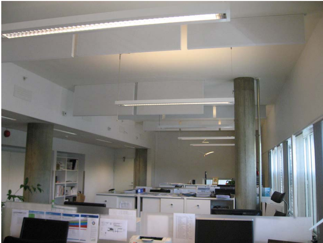
Photo 1. Office building in Prof. Brochs gt. 2 - Open space office area on the third floor, with fair-faced concrete ceilings, hanging acoustic boards and fair-faced concrete pillars (Photo: SINTEF Byggforsk)
