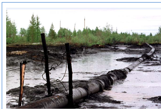
Figure 7: Russian pipeline in thawing permafrost areas ( http://www.desdemonadespair.net/2009/11/permafrost-thaw-threatens-russia-oil.html )
