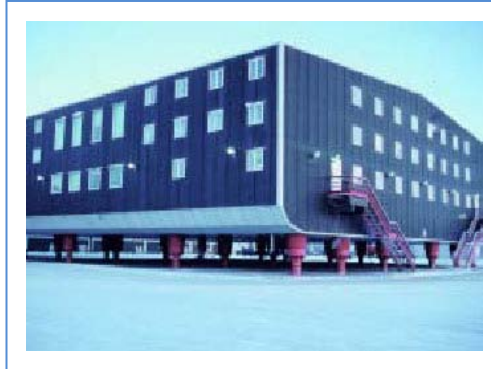
Figure 2: Pillars prevent the building from damage due to thawing permafrost- BP operation center, Prudhoe Bay, Alaska ( www.klimanotizen.de )
