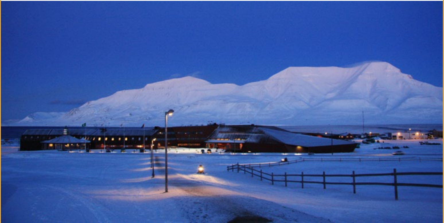
The Svalbard Science Centre. UNIS, the University Centre in Svalbard, occupies the left side of the building complex.
