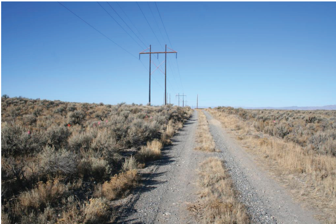
Figure 10. Facing west, general area of site 10-BT-1059, unaffected by range fire.
