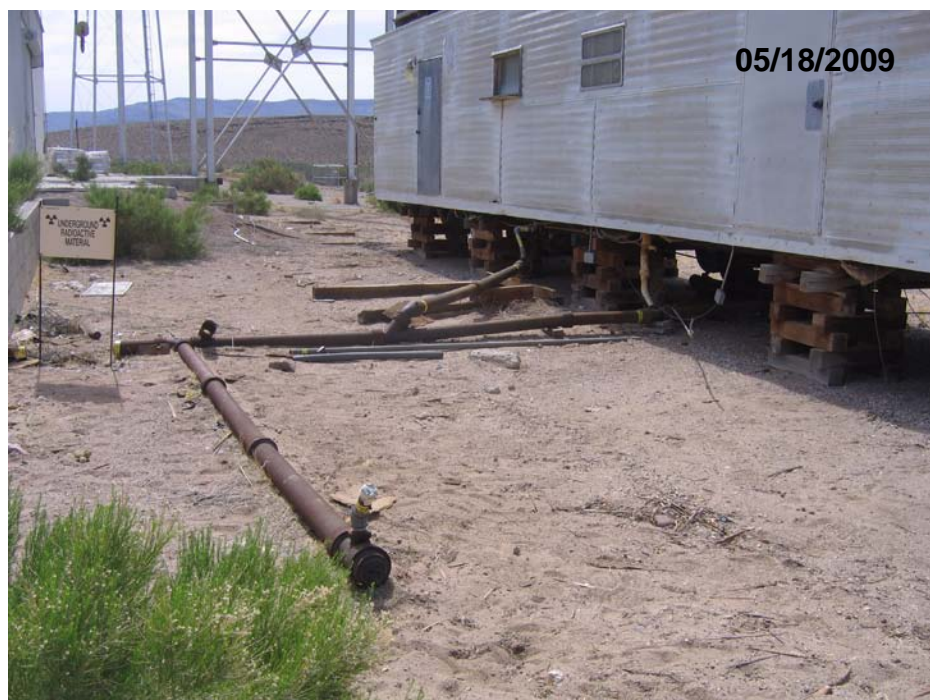
Figure 2-1 Metallurgy Lab Trailer (top) and Drains (bottom)
