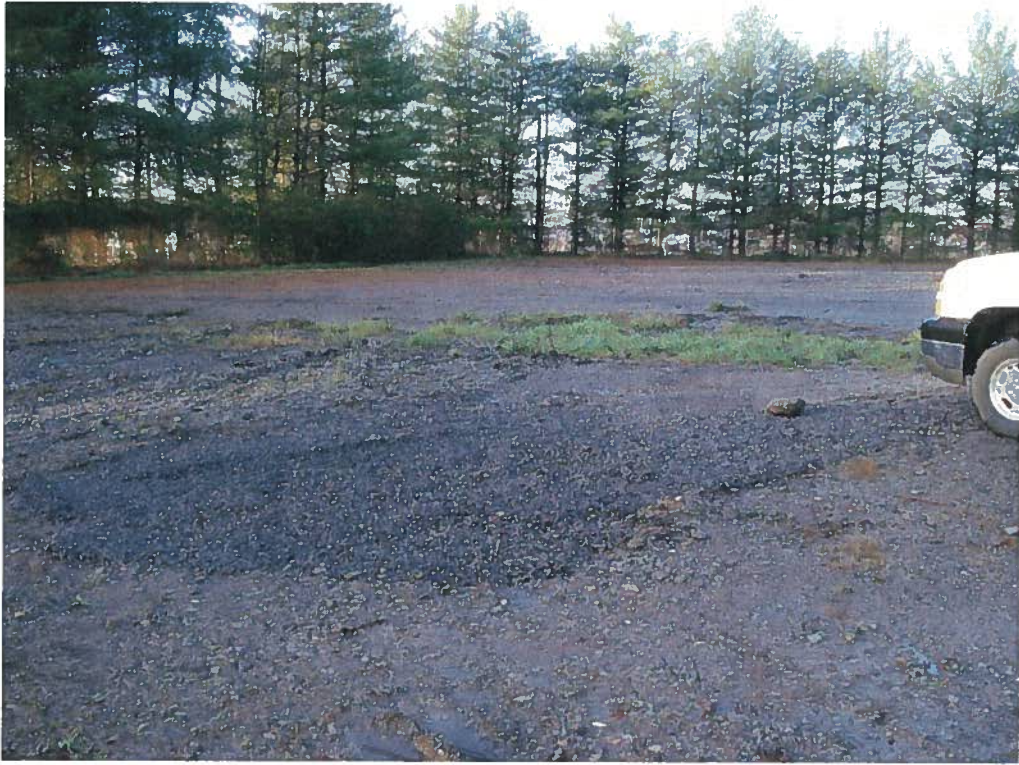
Fig. 7. K-1066-G Yard RA location after excavation backfilling.
