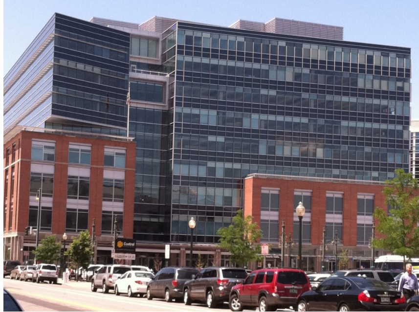
Figure 1: EPA's Region 8 Headquarters Building (Photo by Alicen Kandt, NREL/PIX 19447)
