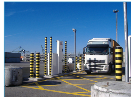
NNSA's Second Line of Defense Megaports Initiative installation of portal monitors at Antwerp in Belgium to detect illicit trafficking of nuclear and radiological material.
