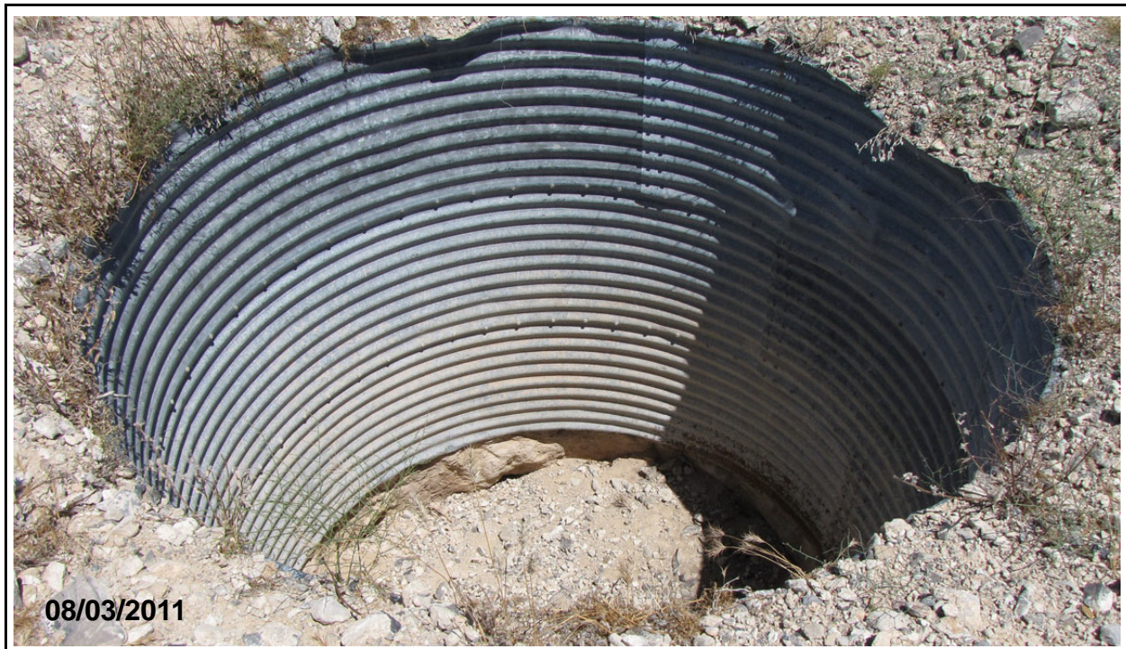
Figure 2-7 Open Disposal Borehole at CAS 00-23-02 (Dog Site)
