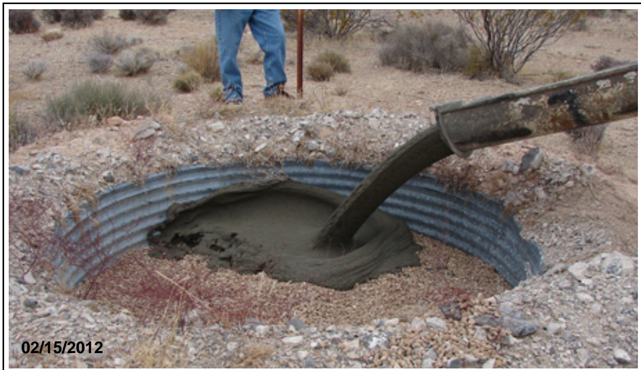
Figure 2-8 Placement of Cement/Sand Slurry at Disposal Borehole at CAS 00-23-02 (Dog Site)
