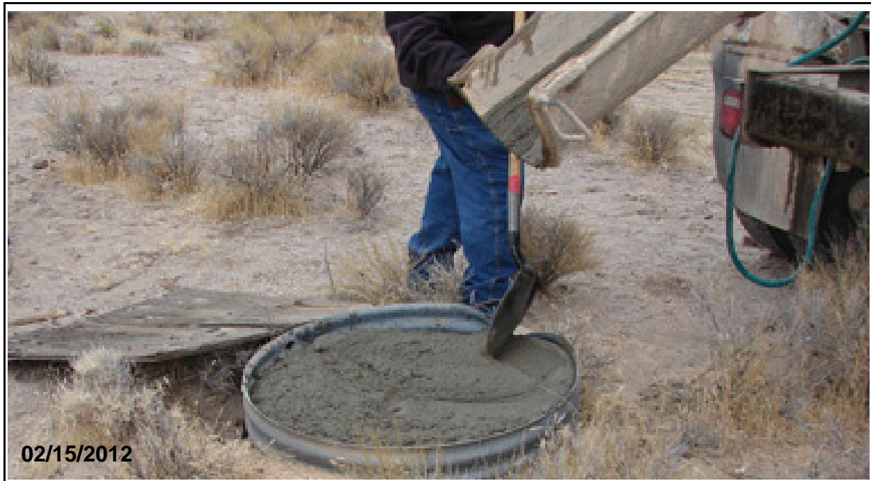
Figure 2-11 Placement of Cement/Sand Slurry at Borehole at CAS 00-23-03 (Anja Site)
