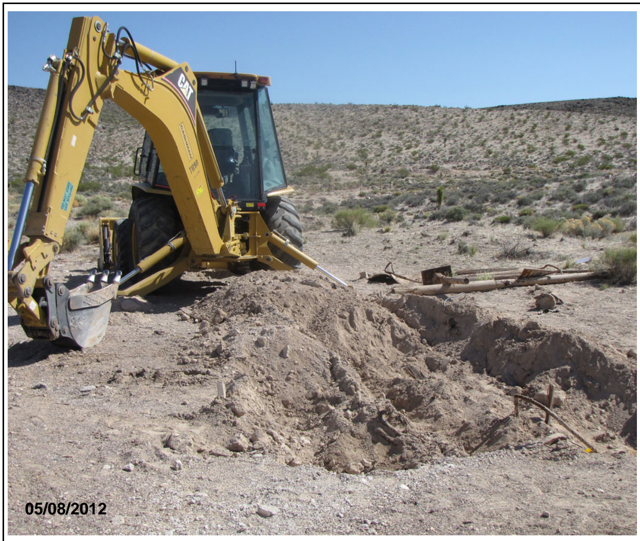
Figure 2-13 Debris Removed from Landfill/Disposal Trench at CAS 00-23-02 (Dog Site)
