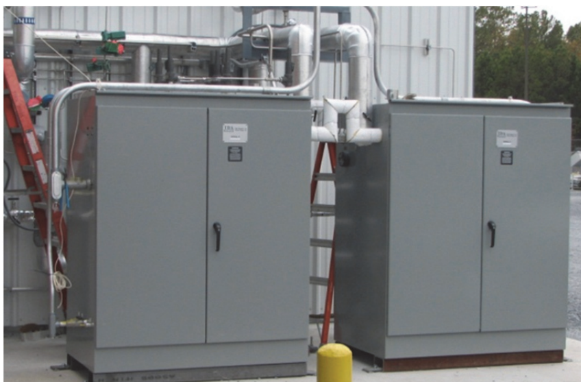
Figure 79. Test Unit Installed At the NCCC.
