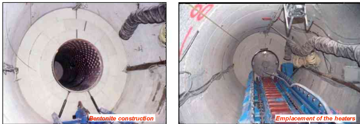
Figure 4-8. FEBEX Test at Grimsel Test Site: Photos taken during the construction phase of the FEBEX test.
