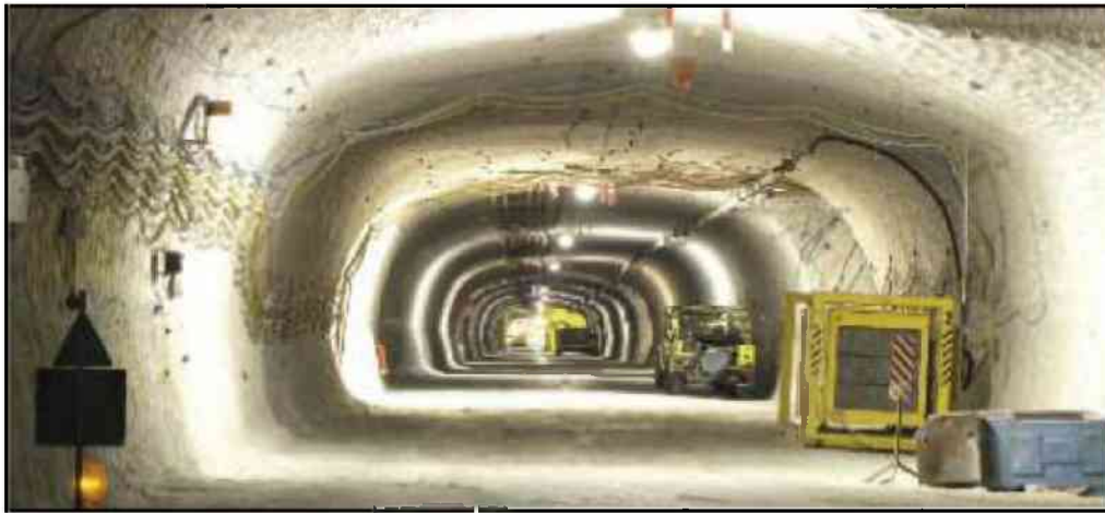
Figure 4-12. View of one of the underground tunnels at Gorleben site at the 840 m level (from BMWi, 2008)
