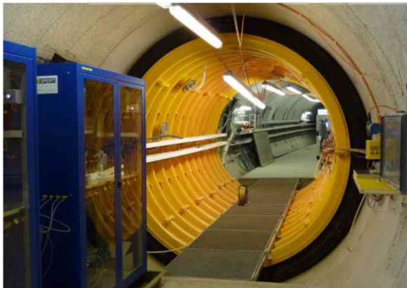
Figure 3-30. CFM field test bed at Grimsel Test Site: Tunnel packer system used to isolate the MI shear zone (from http://www.grimsel.com/gts-phase-vi/cfm-section/cfm-site-preparation ). Small disks with tubing issuing from them (inside yellow packer) are “surface packers” that seal the tunnel wall and collect water from inflow points. Tunnel diameter is 3.5 meters.
