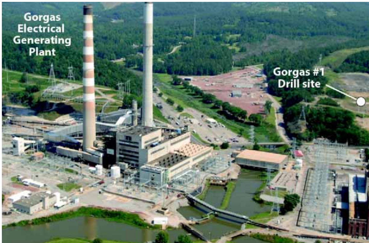
Figure 3.—Photograph of the William Crawford Gorgas Electrical Generating Plant showing location of the Gorgas #1 borehole (photo courtesy of Alabama Power Company).
