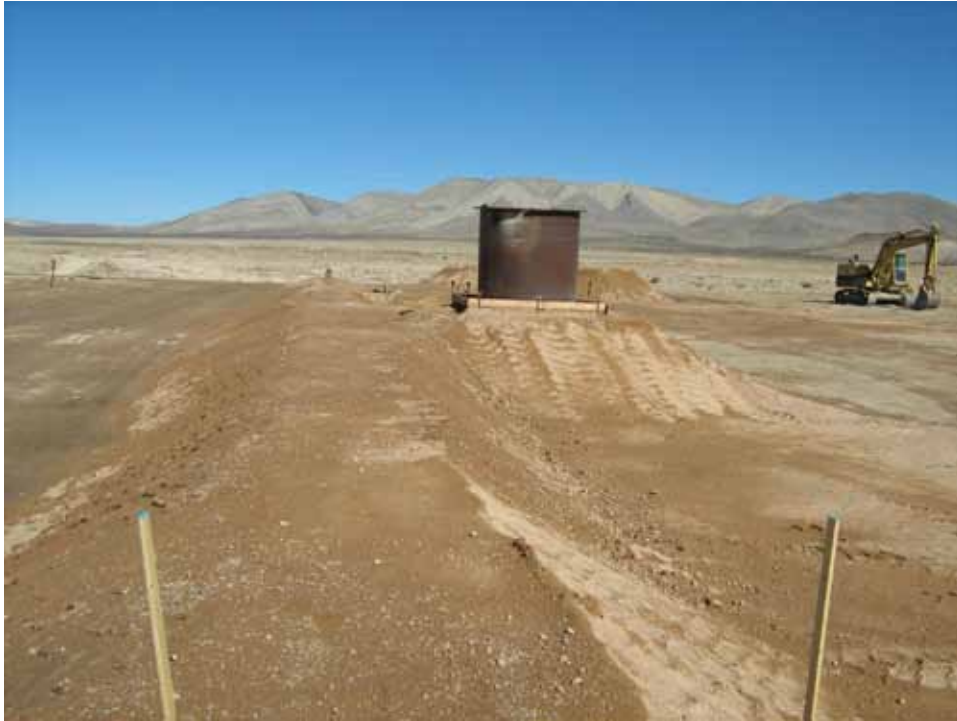
Photograph 35: CAS 09-99-06 (PLAYER), Casing Over Accelerometer and Soil Cover, Looking Northeast, 02/09/2012
