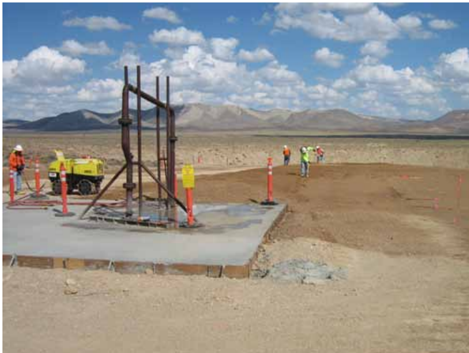
Photograph 6: CAS 02-37-02 (MULLET), Raised and Leveled Concrete Pad, Construction of Soil Cover, Looking East, 09/12/2011
