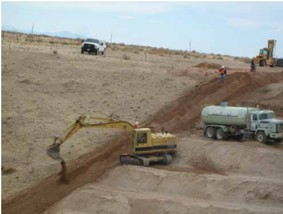
Photograph 42: CAS 09-99-06 (PLAYER), Construction of Soil Cover on YORK Crater Slope, Looking South, 03/14/2012
