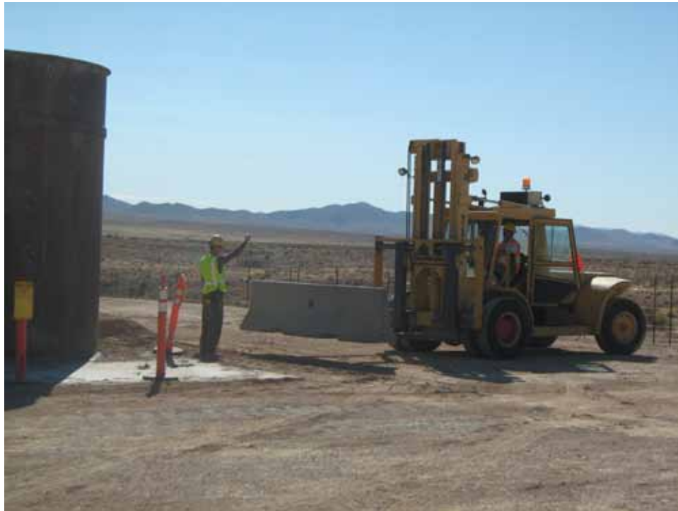
Photograph 9: CAS 02-37-02 (MULLET), Placement of Jersey Barrier, Looking Southwest, 09/26/2011
