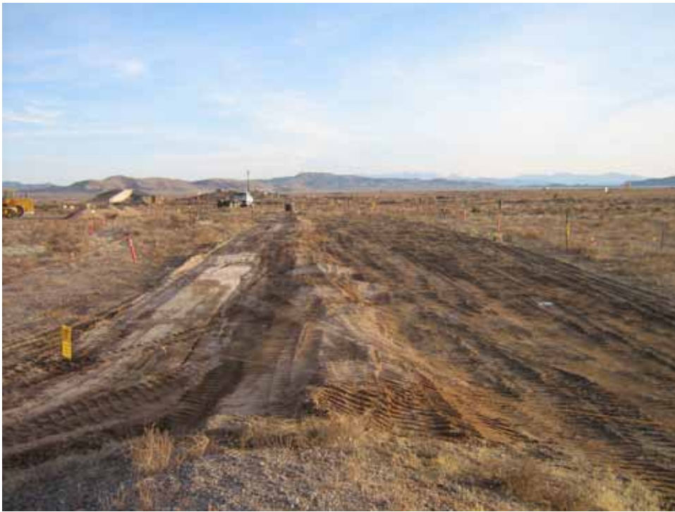
Photograph 18: CAS 03-99-19 (TEJON), Compaction of Soil at TEJON, Looking South, 11/09/2011
