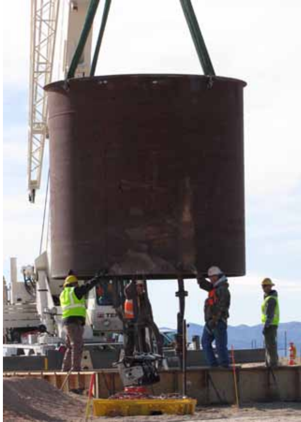
Photograph 33: CAS 09-99-06 (PLAYER), Placement of Casing at PLAYER, Looking South, 02/08/2012
