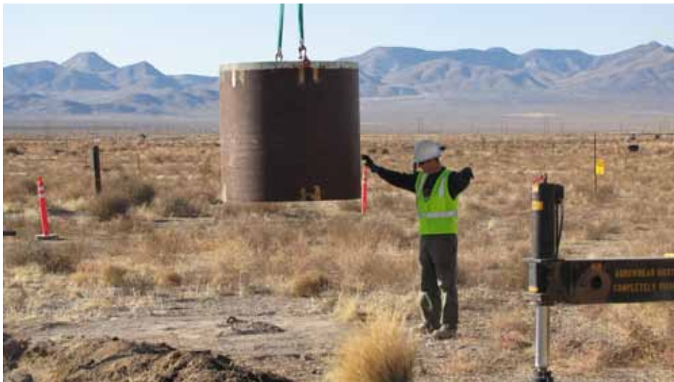
Photograph 16: CAS 03-99-19 (TEJON), Placement of Casing Over the Sampling Can at TEJON, Looking North, 11/08/2011
