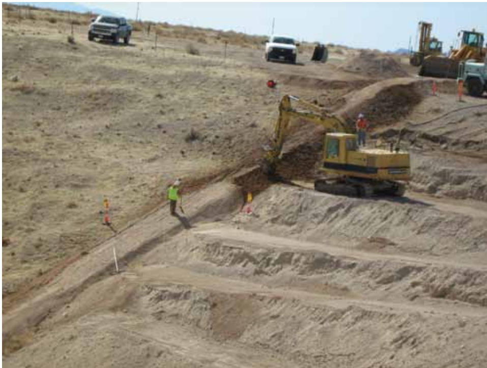
Photograph 40: CAS 09-99-06 (PLAYER), Compaction of Soil Cover on YORK Crater Slope, Looking South, 03/07/2012
