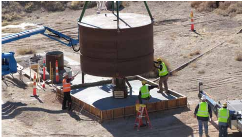
Photograph 34: CAS 09-99-06 (PLAYER), Placement of Casing Over YORK Wellhead, Looking South, 02/08/2012
