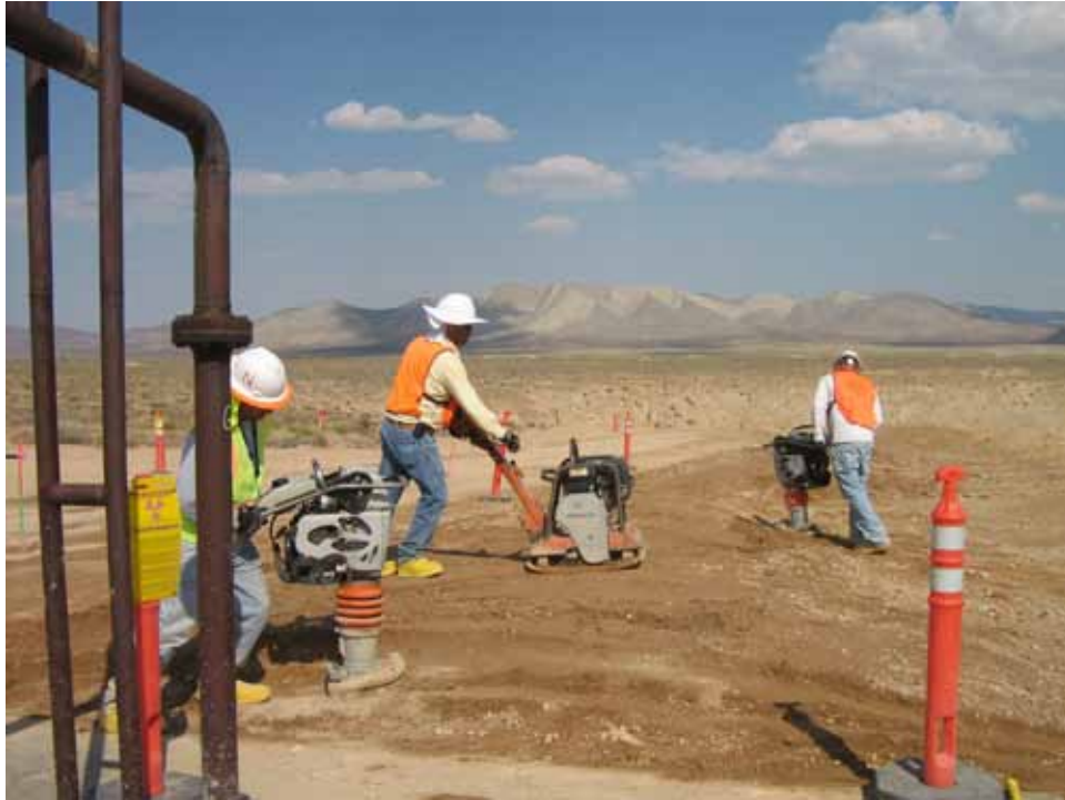
Photograph 5: CAS 02-37-02 (MULLET), Compaction of Soil Cover, Looking East, 09/09/2011
