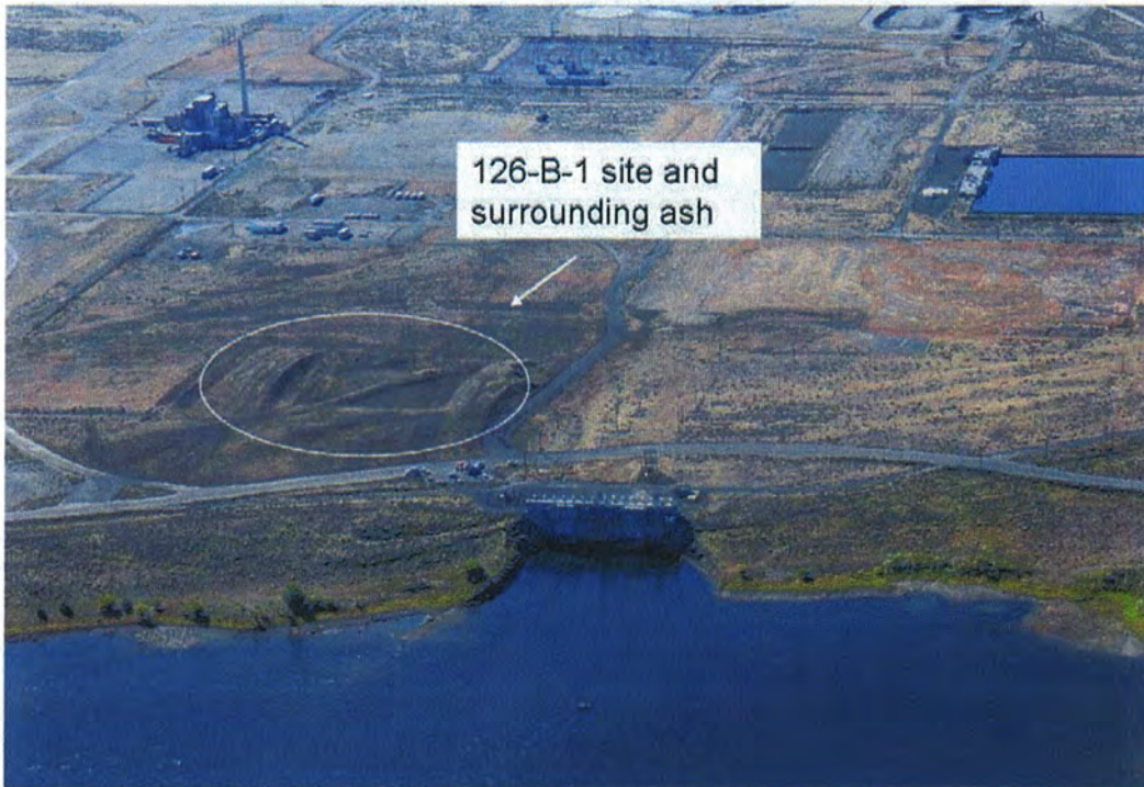
Figure B-1. 126-B-1 Coal Ash Sample Site and Surrounding Coal Ash Area.
