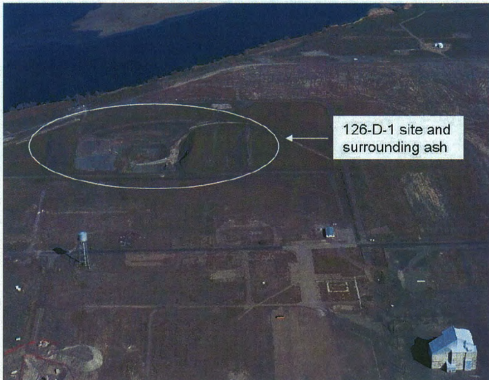
Figure B-4. 126-D-1 Coal Ash Sample Site and Surrounding Coal Ash Area (View to North).
