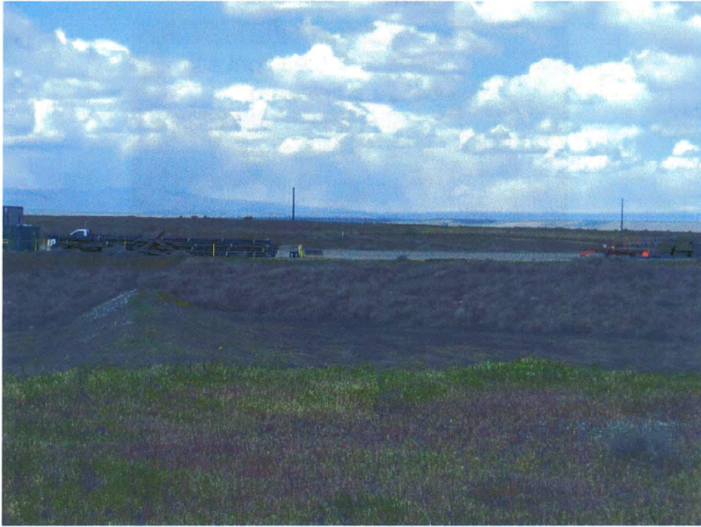
Figure B-9. View to North of Midline Berm at 126-H-1 Site.
