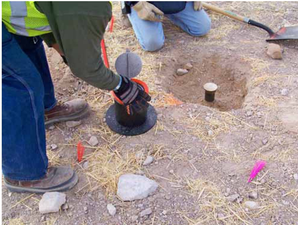
Photograph 12: Installing Subsidence Survey Monument, 01/19/2012
