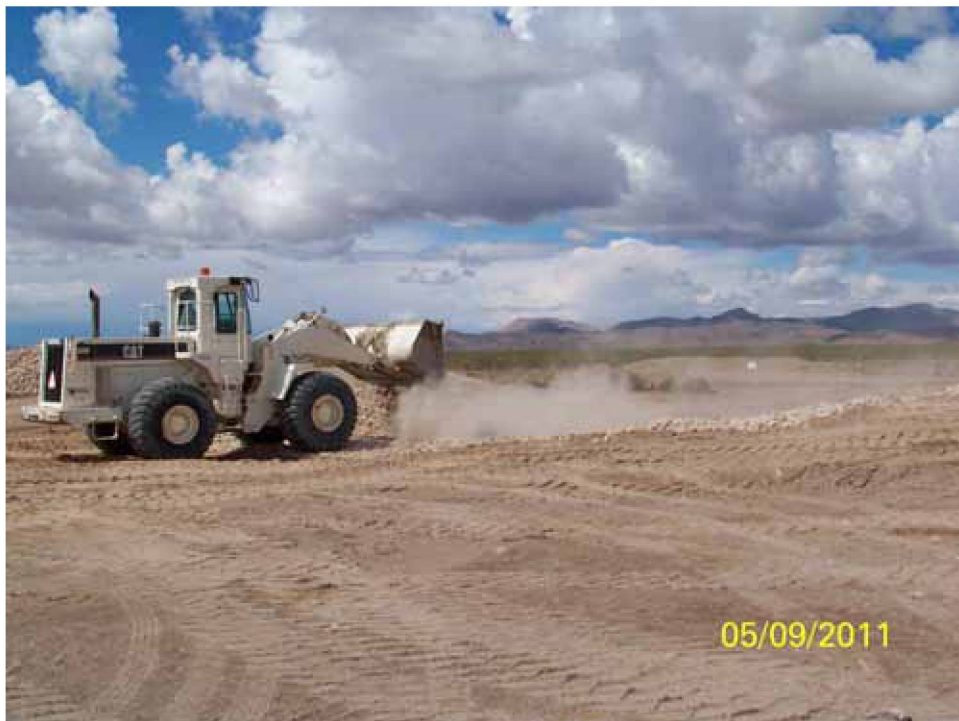
Photograph 8: Placing Riprap in Arizona Crossing, 05/09/2011
