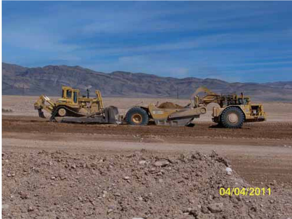
Photograph 3: Loaded Backfill Material for Cover Construction, 04/04/2011
