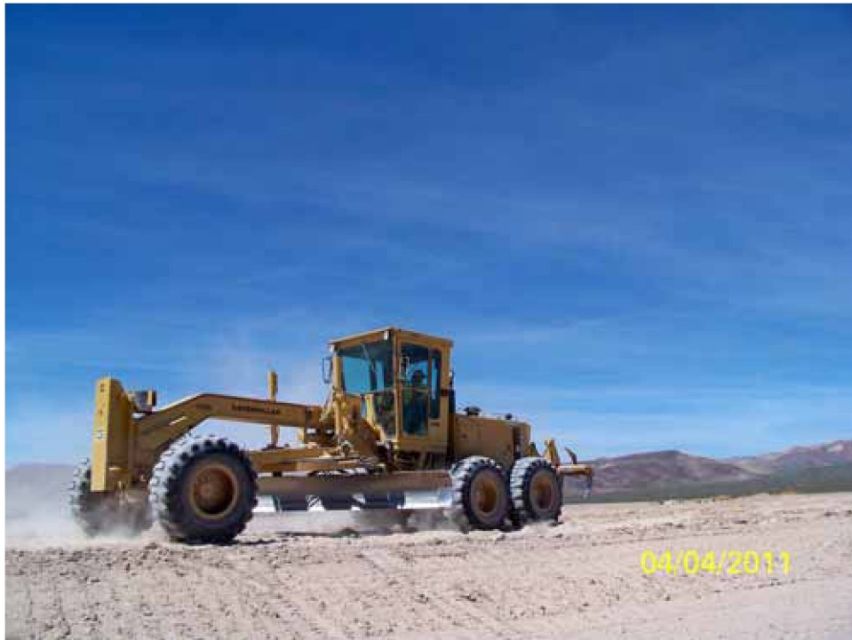
Photograph 4: Equipment Used for Ripping the Cover, 04/04/2011
