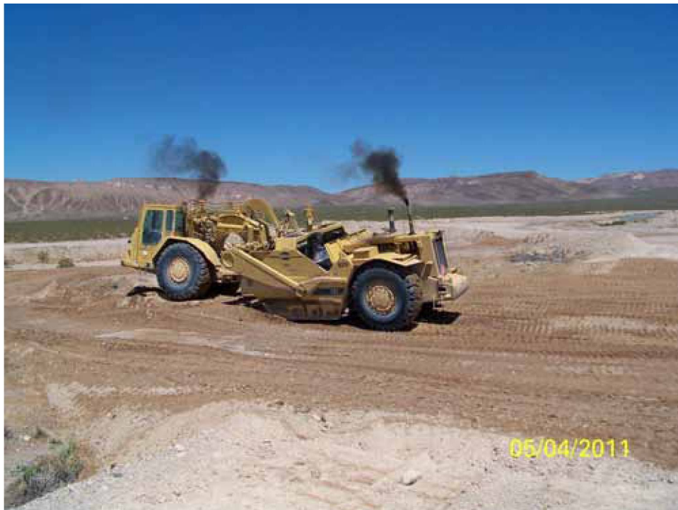
Photograph 6: Placing Cover Material, 05/04/2011
