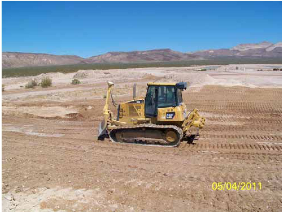
Photograph 7: Ripping the Cover, 05/04/2011
