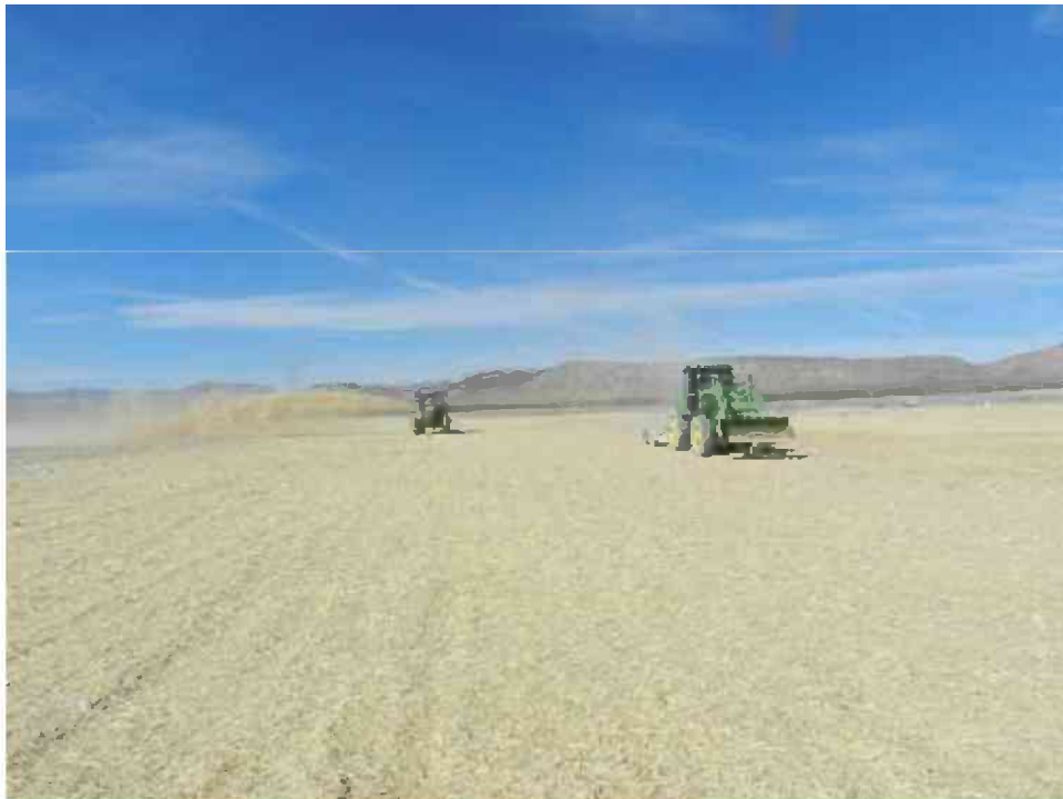
Photograph 10: Installing Straw Mulch and Crimping, 11/03/2011
