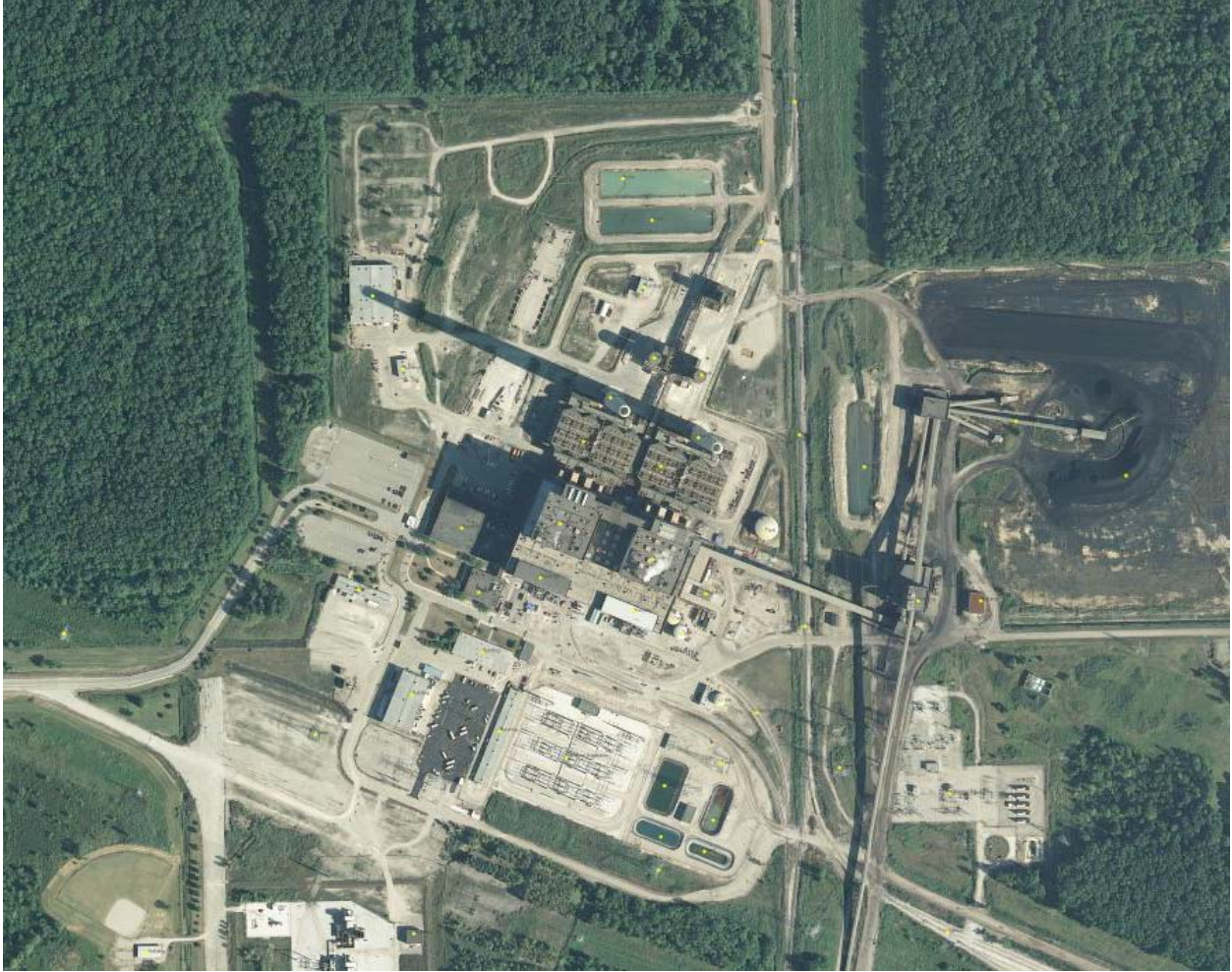
Figure 3. Illustration of a Heat Processing Plant, HP0058_C8, Belle River power plant, a coal-fired plant located in China Township, Michigan, Latitude 42.774676, Longitude -82.494964, GSD: 0.3m.
