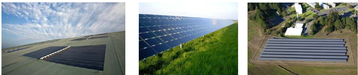
Figure 4. Thin-film solar panels installed on (left) solar energy cover and (middle/right) fixed-tilt mounting system. Photos from (left) Republic Services, Inc., NREL 23817, (middle) Beck Energy, NREL 14726, and (right) U.S. Coast Guard Petaluma site, NREL 17395
