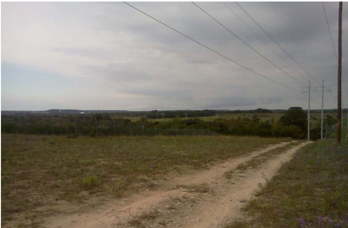
Figure 10. Ground view of the area evaluated for ground-mounted PV at the West Ft. Hood site. Photo by Jesse Geiger, NREL
