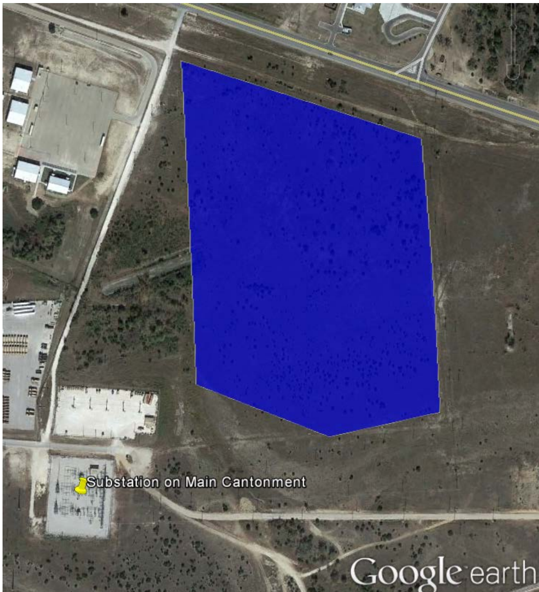
Figure 11. Location of onsite substation near the MC area evaluated for a ground-mounted system
