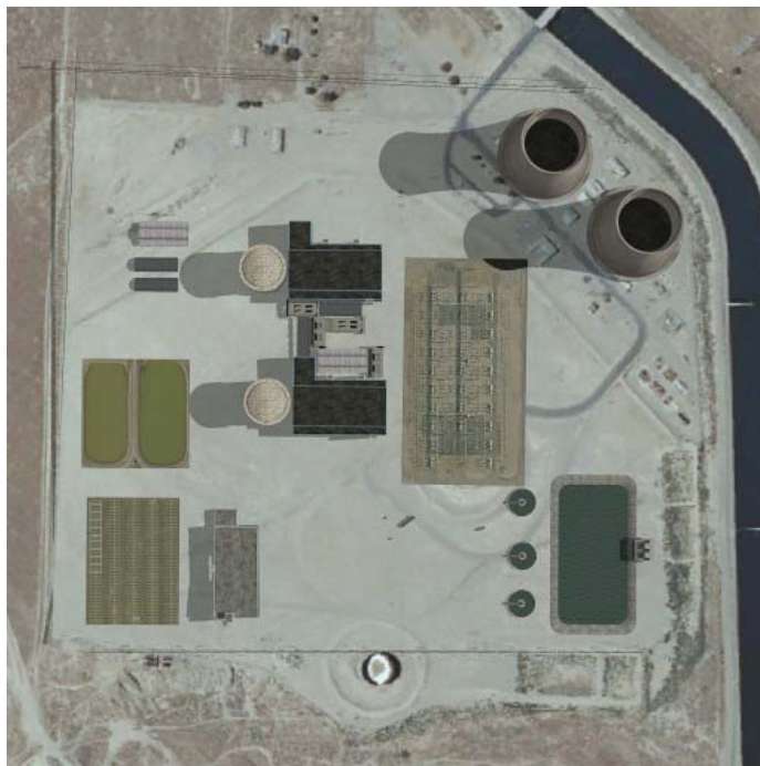
Figure 5 - Synthetic nuclear power plant in arid environment based on layout in figures 3 and 4.
