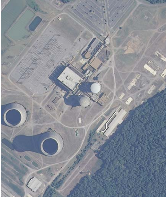
Figure 3 - Bellefonte Nuclear Plant (HP104)
