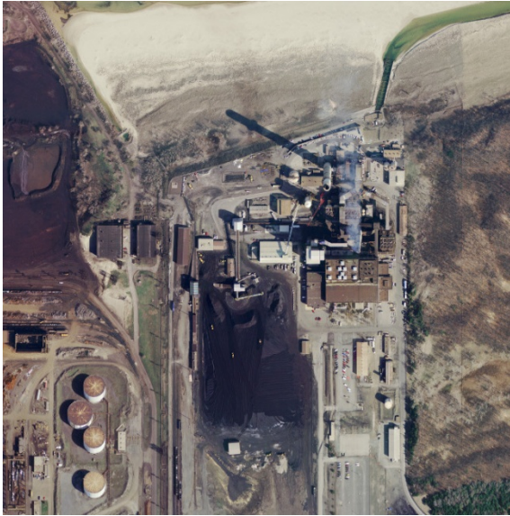
Figure 1 - Bailly Generating Station (HP52)
