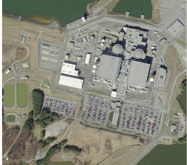
Figure 4 - Duke Energy Mcguire Nuclear Station (HP119)
