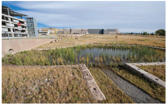
A new stormwater detention pond controls the flow of runoff from much of the STM site and serves as an important local habitat. Photo by Dennis Schroeder, NREL 23195
