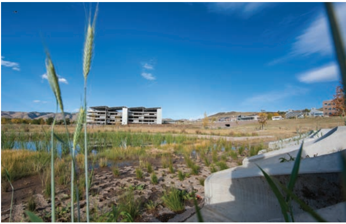
The new stormwater detention pond regulates the flow of runoff from the STM campus and improves water quality. Photo by Dennis Schroeder, NREL 23189
