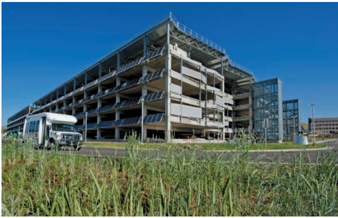
The parking structure on NREL's STM campus includes 3,632 photovoltaic panels installed on the roof and the south façade. The panels produce up to 1.15 megawatts of power. Photo by Dennis Schroeder, NREL 21635
