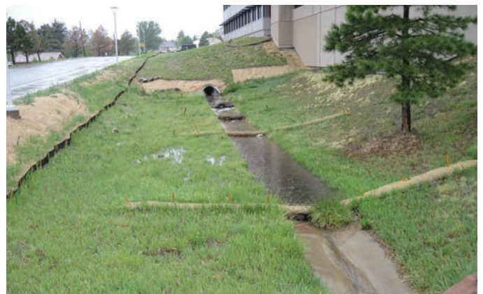
Stormwater best management practices in action at the STM site. Photo by Genny Braus, NREL 24483
