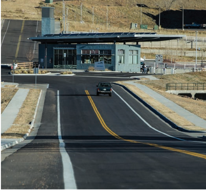
The new South Site Entrance Building on NREL's STM campus is energy efficient, constructed mostly with recycled materials and features a passive cooling tower. Photo by Dennis Schroeder, NREL 23232
