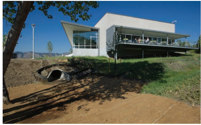
Stormwater erosion control matting at the cafeteria at the STM site. Photo by Dennis Schroeder, NREL 22488
