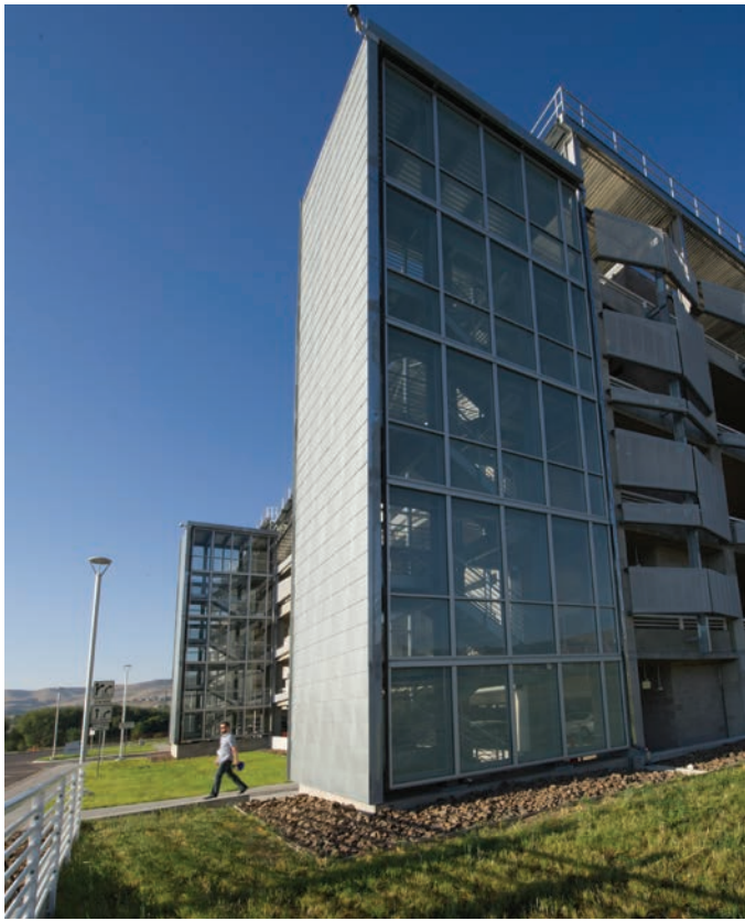
Windows at the parking garage use fritted glass to prevent bird collisions. Photo by Dennis Schroeder, NREL 22479
