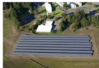
Source: NREL PIX 17395
