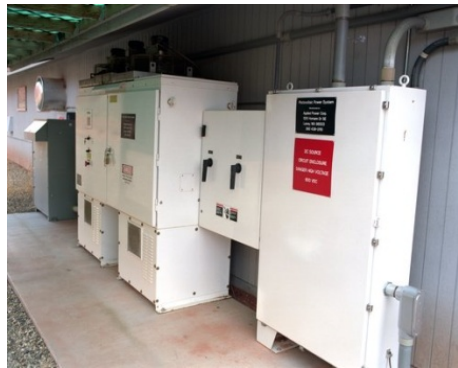
Figure 3-5: String inverter
