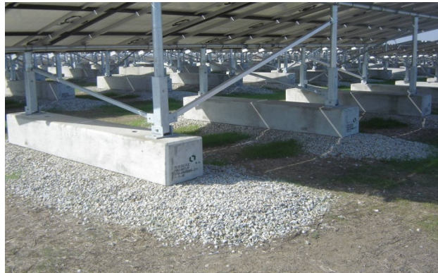
Figure 5-1: Precast ballast foundation for fixed tilt PV on a landfill
