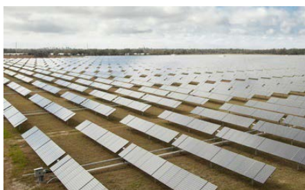
Source: SunPower Corporation
