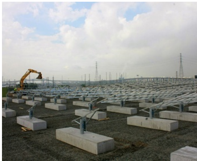
Figure 5-3: Ballasted anchoring system at Landfill 1A project at New Jersey Meadowlands
