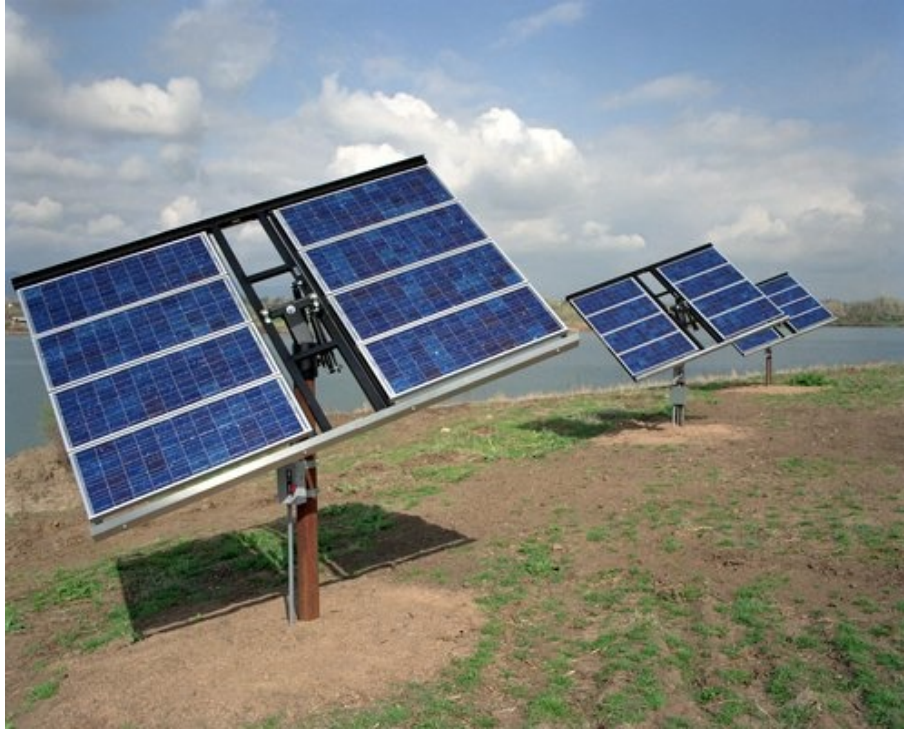
Figure 3-8: PV system with dual-axis trackers
