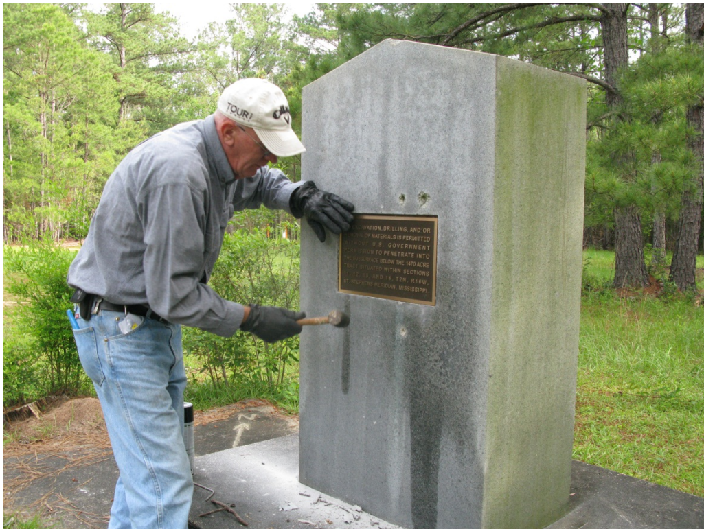
Image A-2. Installing the new bronze plaque on the monument.
