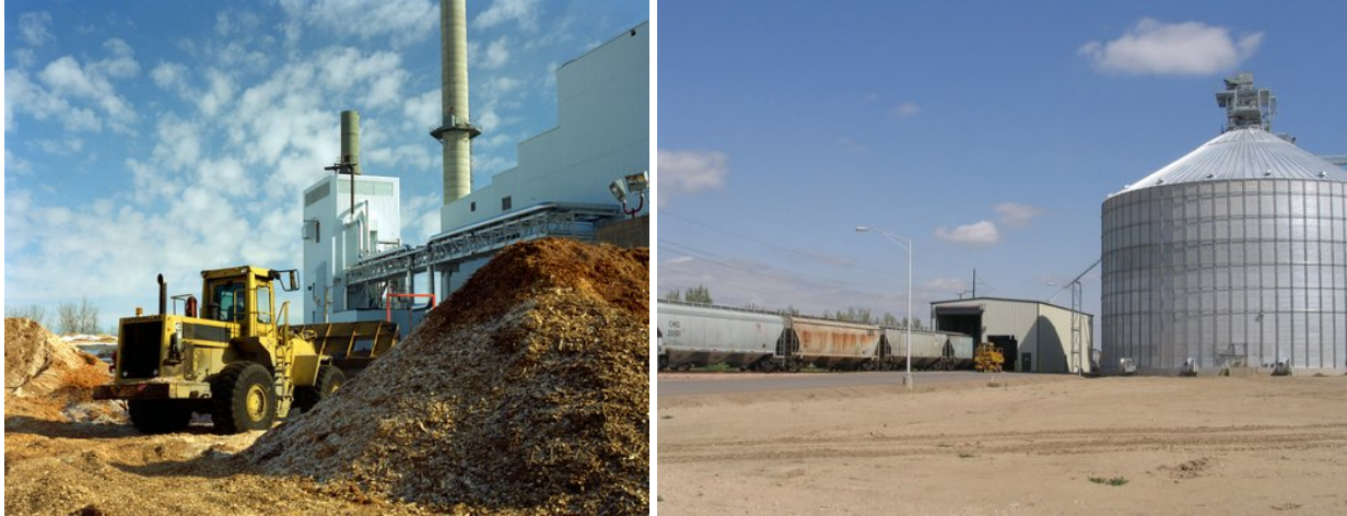
Figure 9. Biomass storage options: fuel yard (left) and fuel silo (right). Photos by Warren Gretz, NREL 04736 (left) and Gerry Harrow, NREL 15041 (right)
