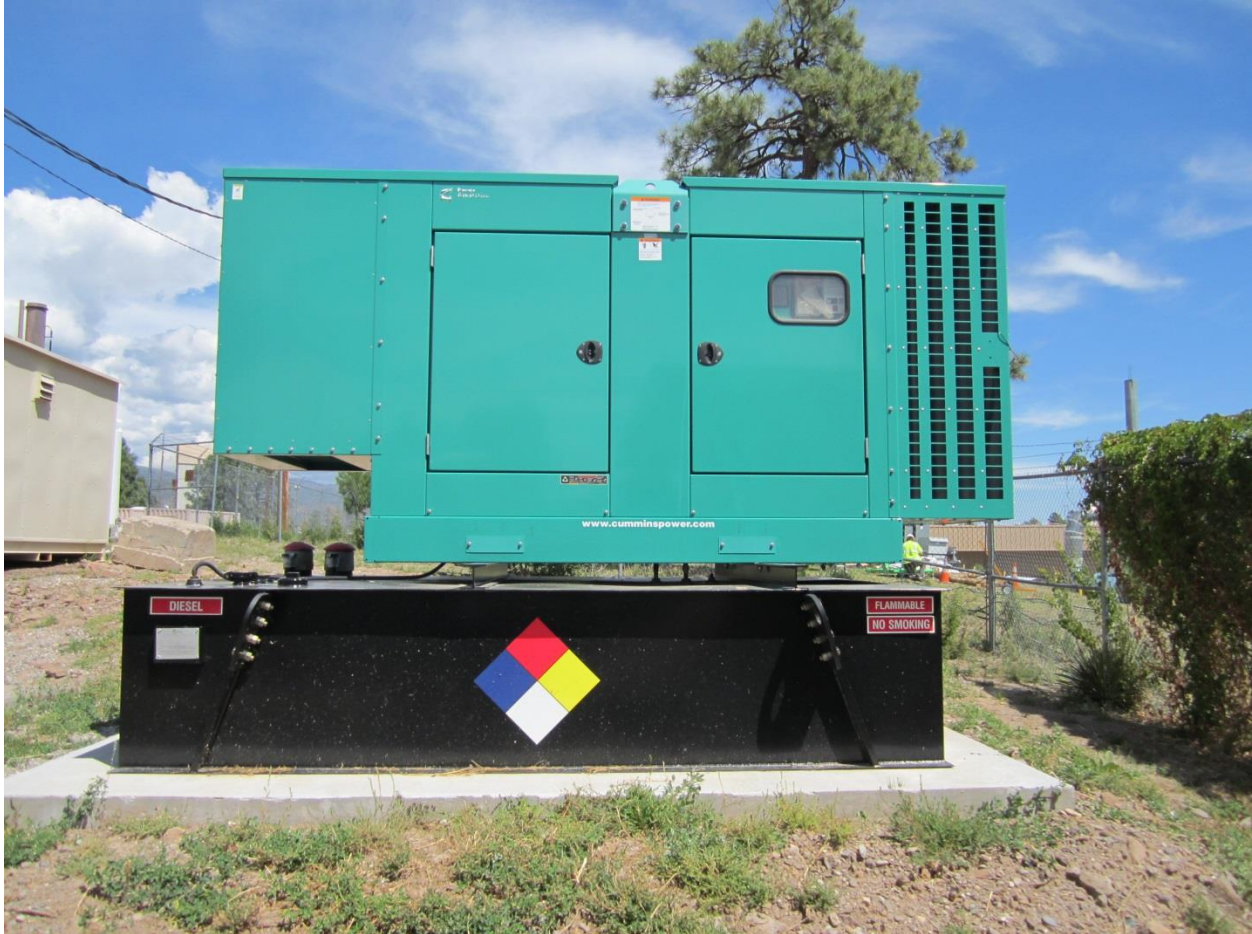
Figure 2: RC-1 Generator and Associated Aboveground Storage Tank
