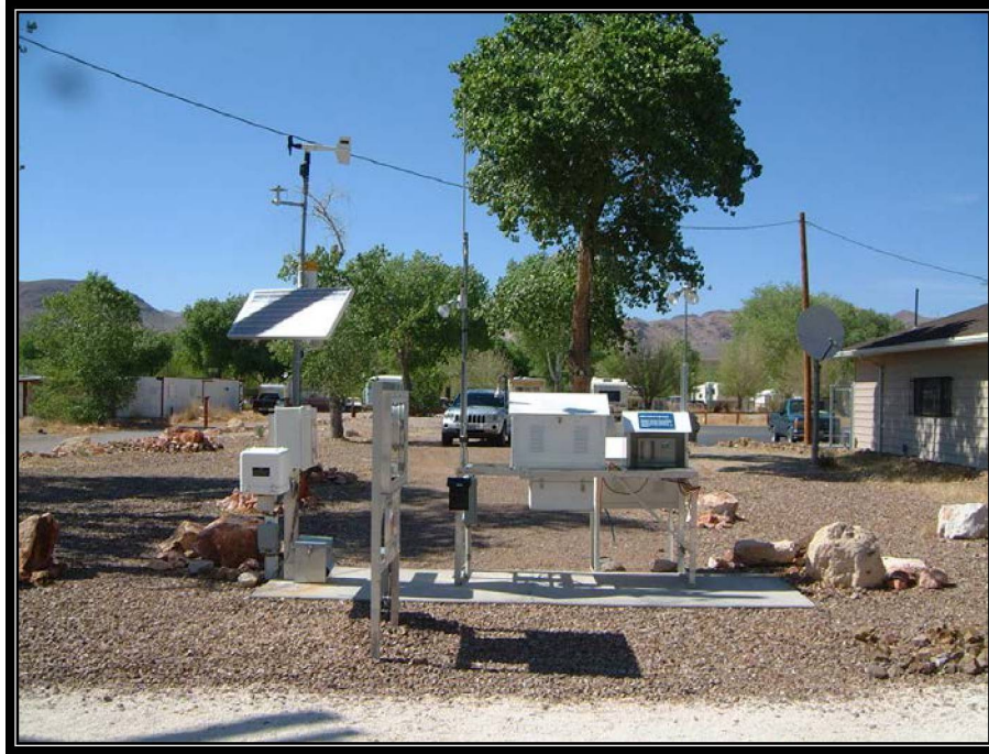
Figure 7-2. CEMP Station in Beatty, Nevada
