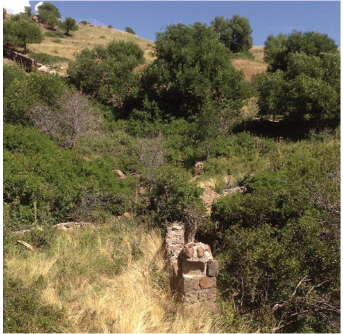
Remnants of a stone bridge located on the STM campus. Photo by Kurt Schlomberg, NREL 33061
