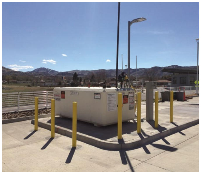
E85 fuel tank and fueling station at the STM campus. Photo by Larry Durbin, NREL 32761
