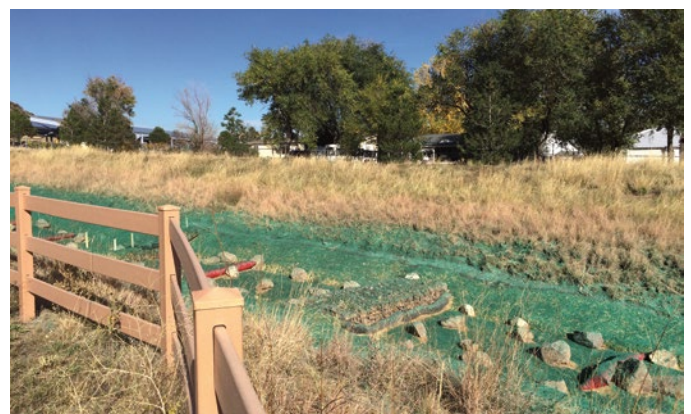
Improvements and erosion control measures at the Jeffco Swale. Photo by Karri Bottom, NREL 32736
