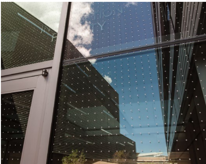
Energy Systems Integration Facility main entrance windows after a special film was applied to help prevent bird collisions. Photo by Dennis Schroeder, NREL 31185
