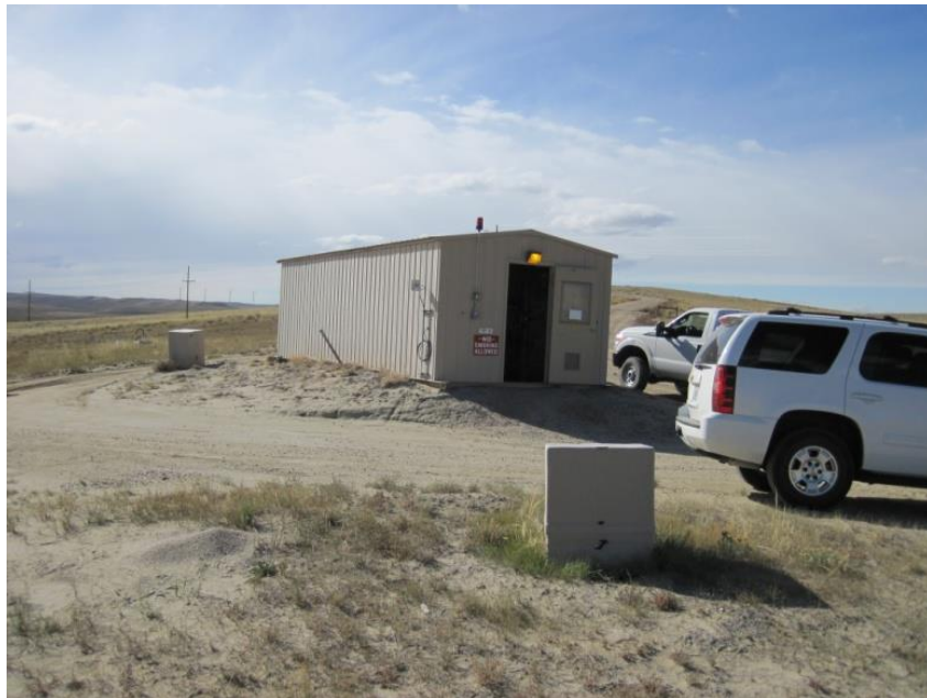
Figure A-2. Close up view of Header House 4-6.
