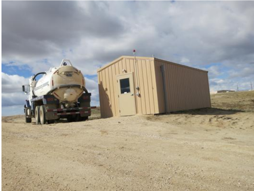
Figure B-1. Header House 7-5, October 2014.
