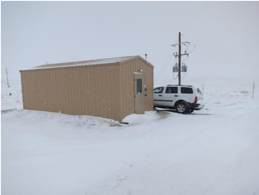
Figure B-2. Header House 7-5, January 2015.
