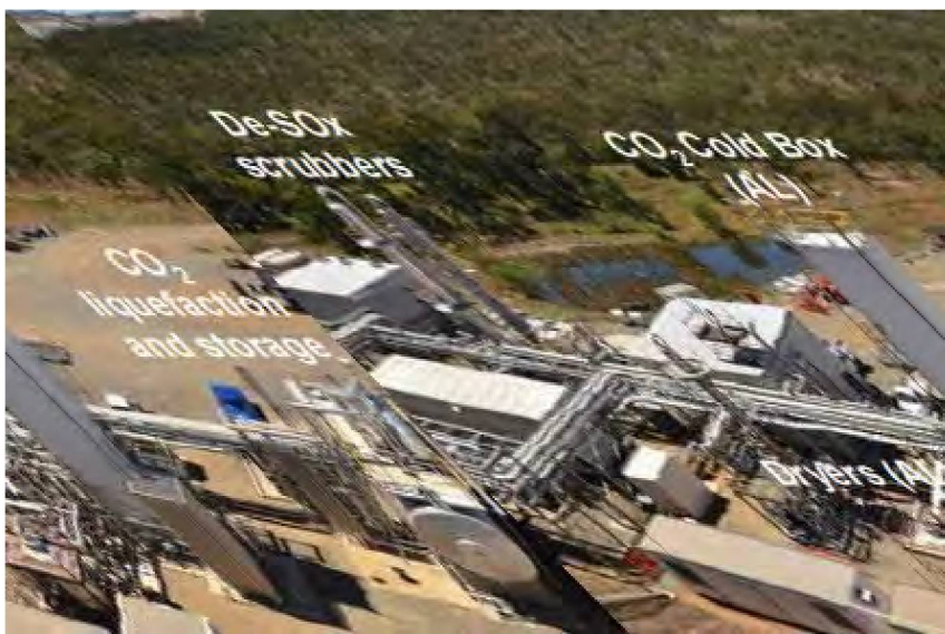
Figure 3-44: Callide Pilot Plant - Site View, September 2011
