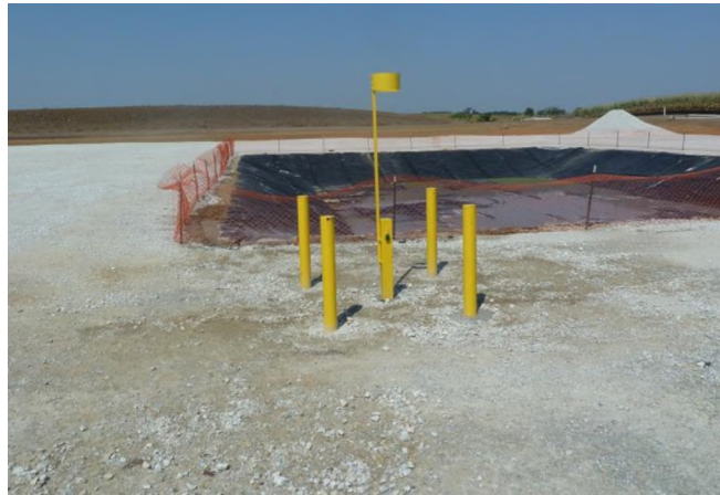
Figure 4.23. Shallow-Well Surface Completion
