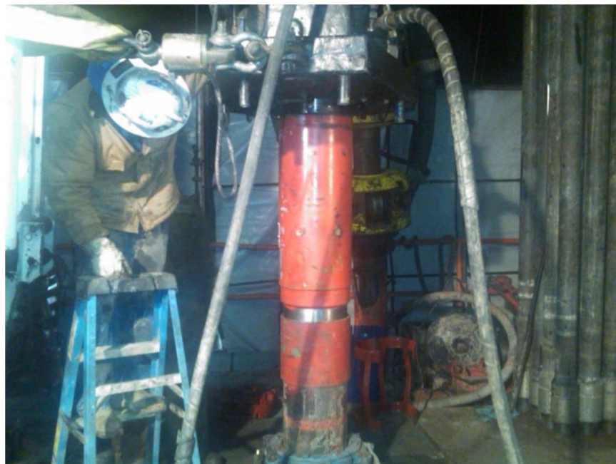
Figure 4.27. Installation of the 10 3/4-in. Multiple-Stage Cementing Collar
