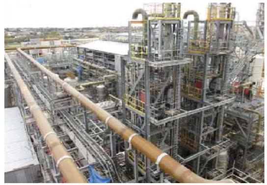
Figure 12 Flue Gas Ducts and HCl Synthesis Units
