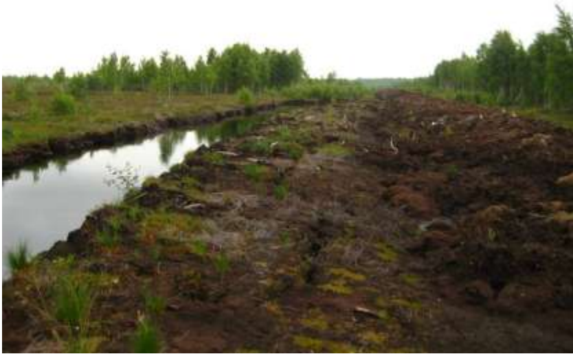
Figure 8: Blocked lateral draining channels and main reservoir (G. Anzaldua)
