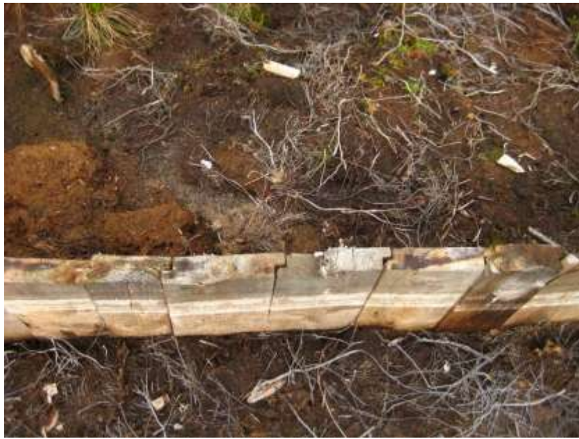
Figure 6: Wooden dam reinforced with peat and impermeable material (G. Anzaldúa)
