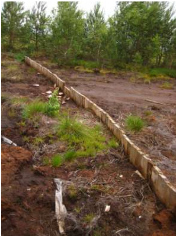
Figure 5: Wooden dam reinforced with peat and impermeable material (G. Anzaldua)
