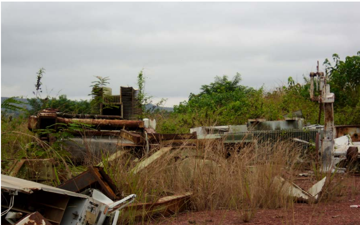
Exhibit 4: Remains of the uranium processing facility in Mounana, Gabon.
