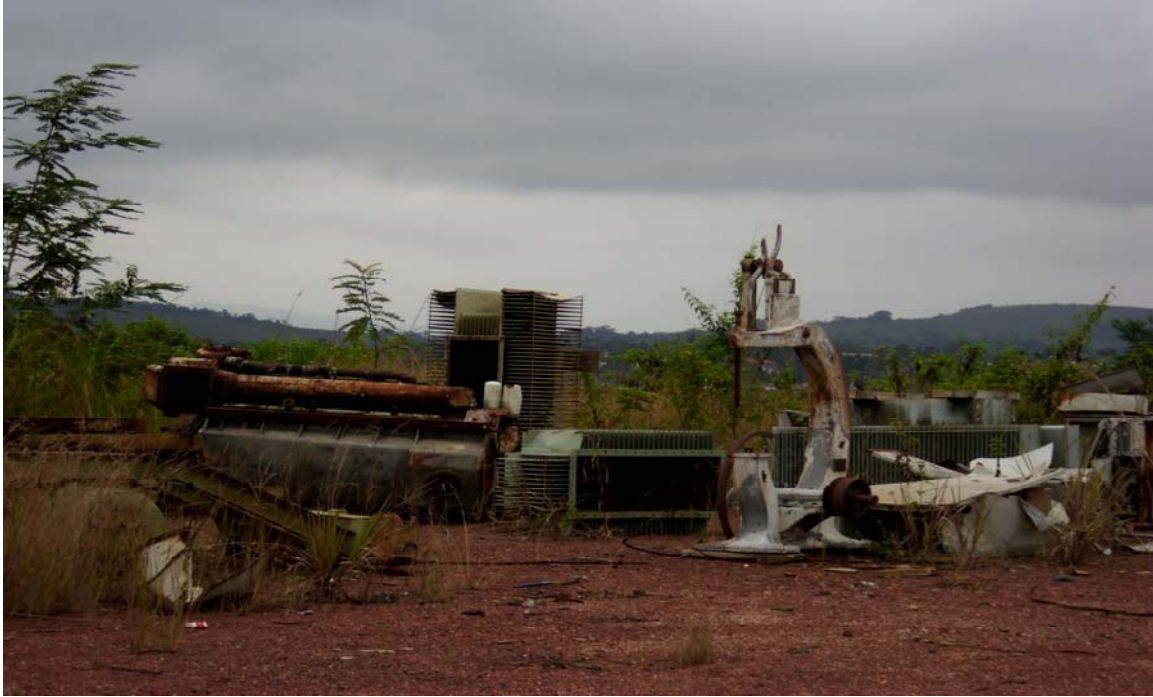
Exhibit 3: Remains of the uranium processing facility in Mounana, Gabon.
