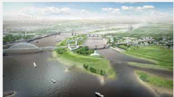
Photo: © Municipality of Nijmegen
