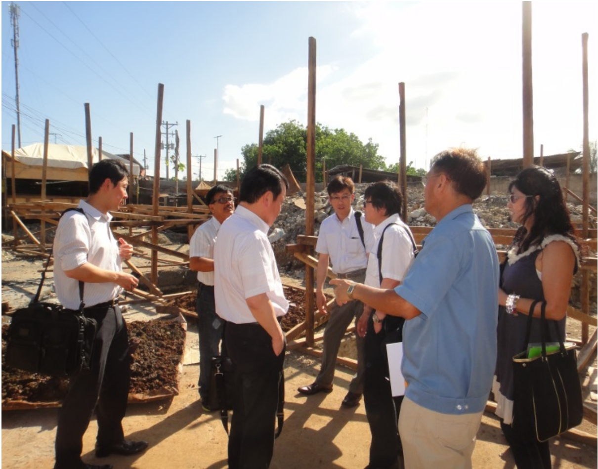
Figure 17: An e-waste treatment facility under construction Source: Author, 2015
