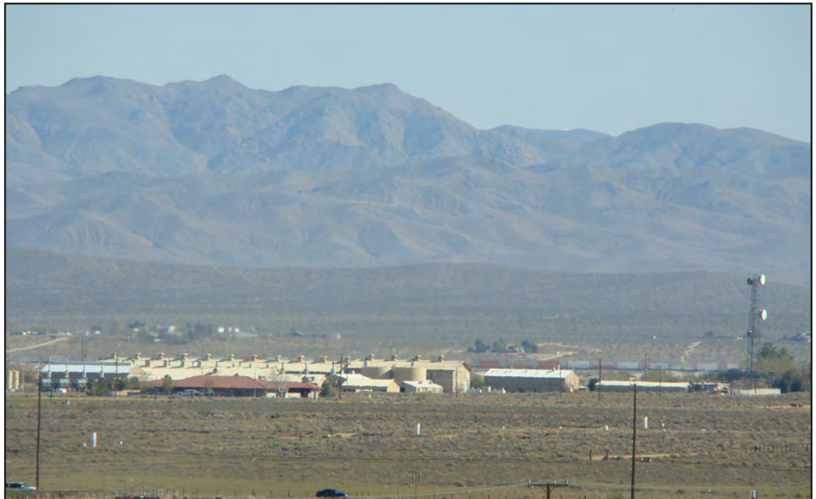
Figure 1. Pacific Gas and Electric (PG&E) compressor station, Hinkley, California, March 2009. (Photo by Steven Perry, Arcadis, Inc., courtesy of PG&E).
