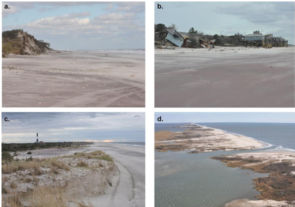
Figure 2. Photos of Fire Island 2 to 4 days after Sandy made landfall: a) leveled beaches and scarped dunes in central Fire Island; b) houses undermined and destroyed at Davis Park; c) leveled dunes and large overwash sheets near Fire Island lighthouse; and d) the island breach at Old Inlet.
