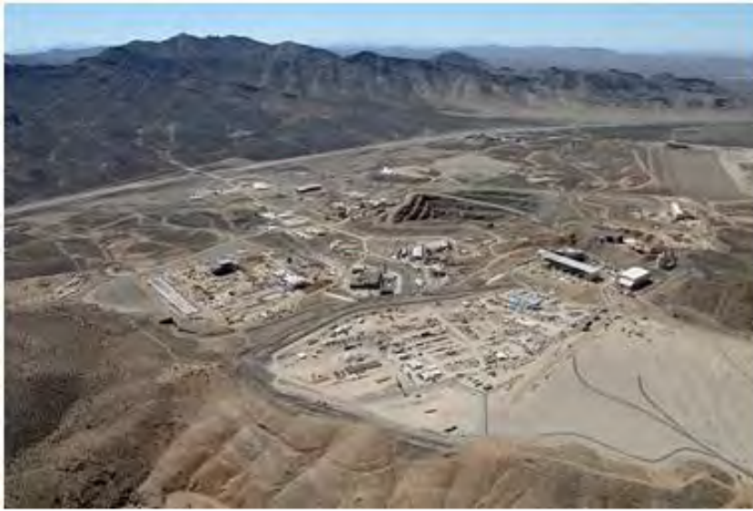
Figure 2. Aerial photograph of Molycorp, Inc.'s Mountain Pass rare-earth oxide mining and processing facilities in Mountain Pass, California. Photograph courtesy of Molycorp, Inc., used with permission.
