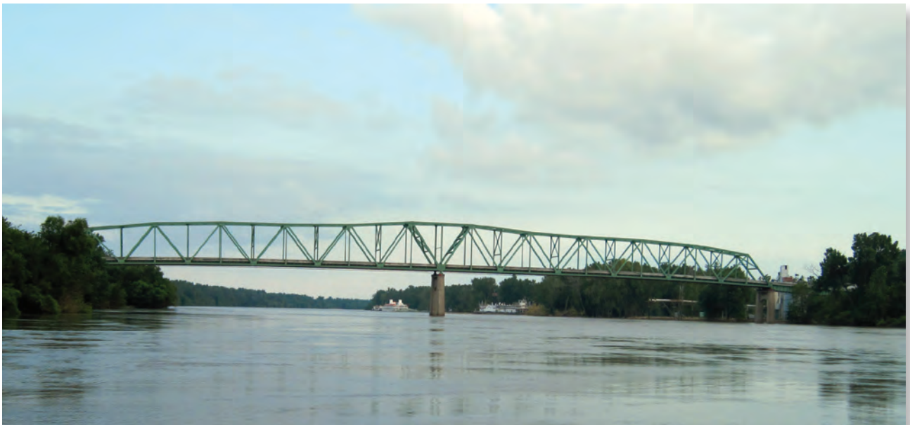
Structure L0098 on U.S. Highway 136 at Brownville, Nebraska.
