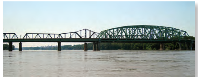
Dual bridge structure A4557 on State Highway 370 near St. Louis, Missouri. The Wabash railroad bridge is in the background.
