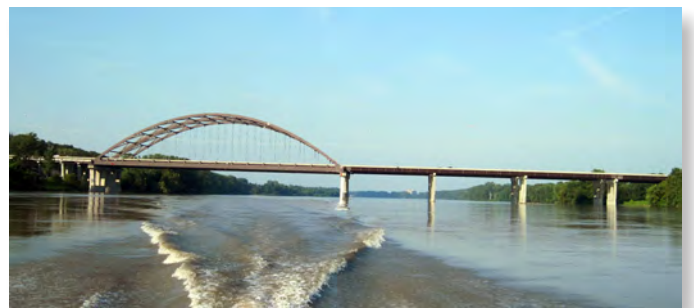
Dual bridge structure A5585 on State Highway 364 near St. Louis, Missouri.
