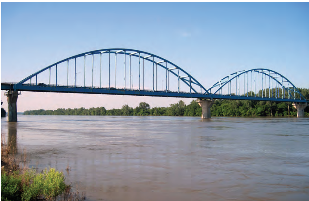
Structure 92-52-18.48 (026) on State Highway 92 at Leavenworth, Kansas.
