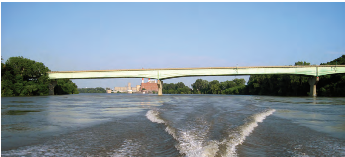
Structure A1800 on Interstate 635 in Kansas City, Missouri.
