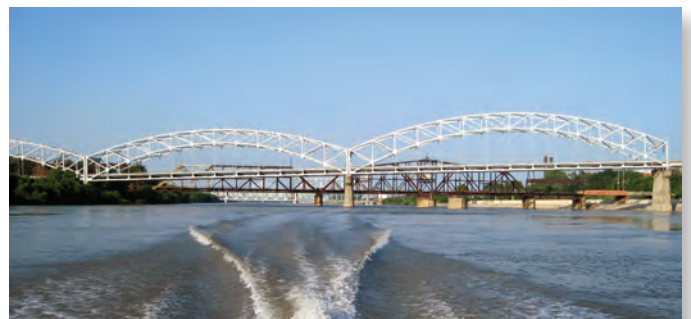
Structure A4649 on U.S. Highway 169 in Kansas City, Missouri. The second Hannibal railroad bridge is in the immediate background.
