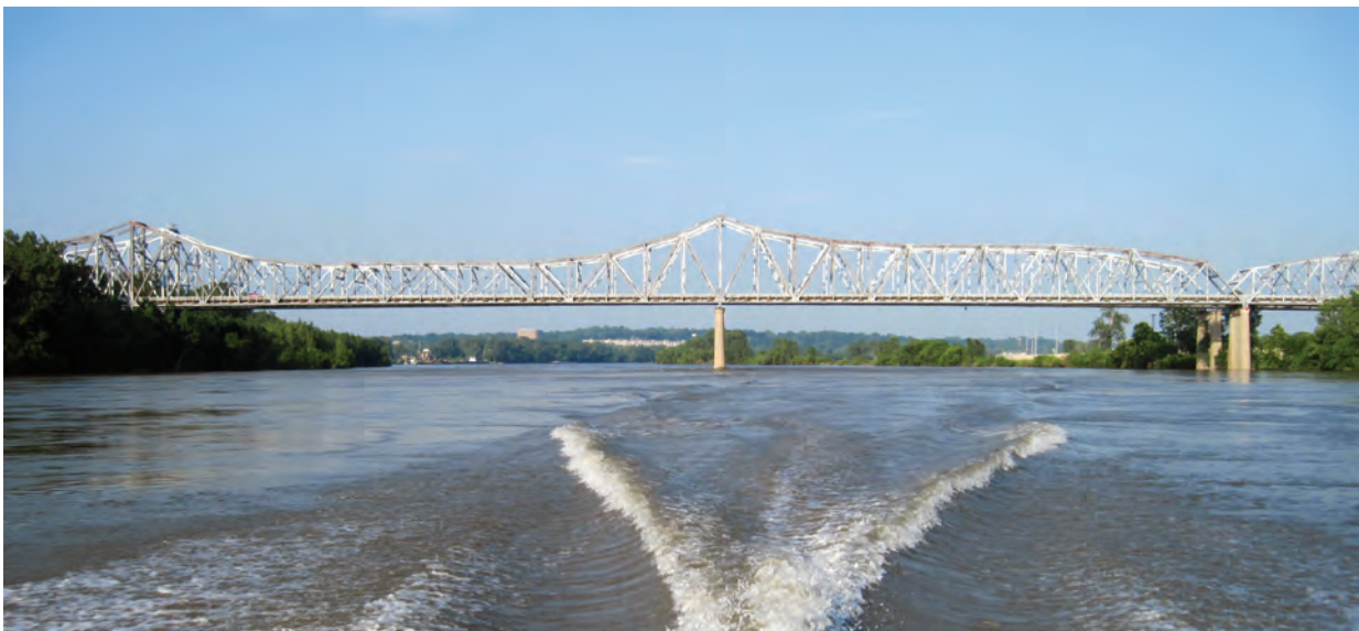
Structures K0456 and A0450 on U.S. Highway 69 in Kansas City, Missouri. Structure K0456 is in the foreground and A0450 is in the background.
