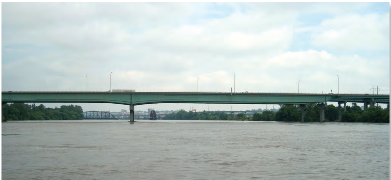
Dual bridge structure A3664 on U.S. Highway 36 at St. Joseph, Missouri.
