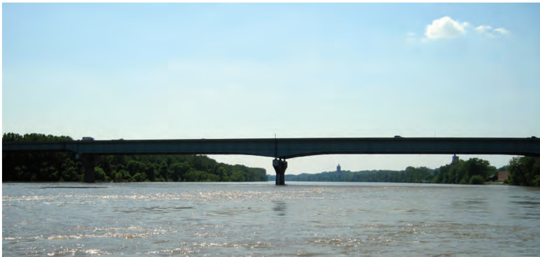
Structure A0767 on Interstate 435 in Kansas City, Missouri.
