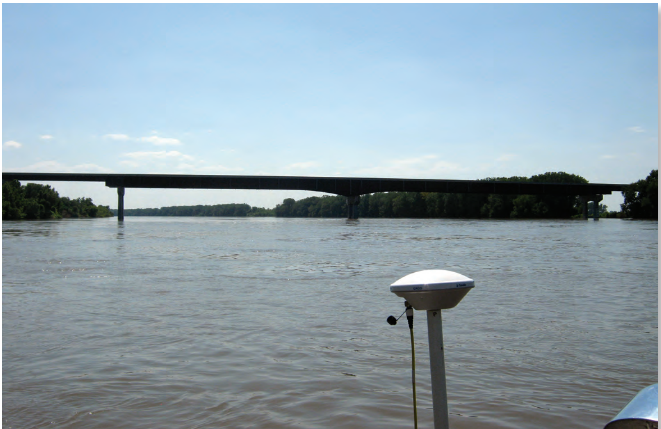
Structure A5664 on State Highway 13 at Lexington, Missouri. Photograph by Joseph Richards, USGS.
