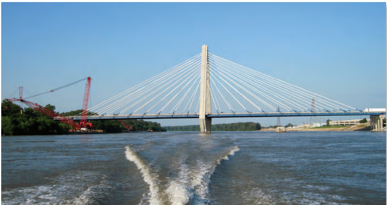
Structure A7650 on Interstate 35 in Kansas City, Missouri.
