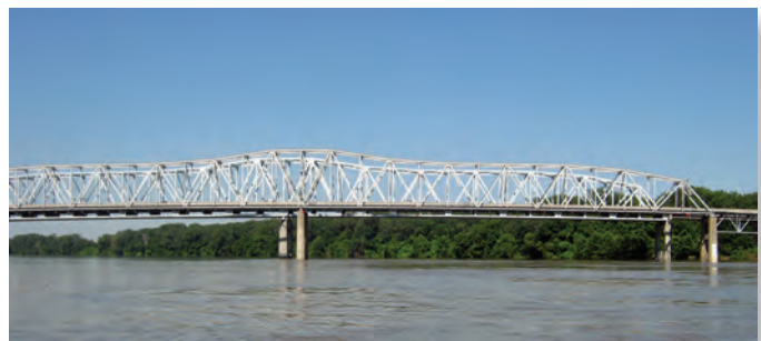
Structures A4757 and L0568 on State Highway 291 in Kansas City, Missouri. Structure L0568 is in the foreground and A4757 is in the background. Photograph by Joseph Richards, USGS.
