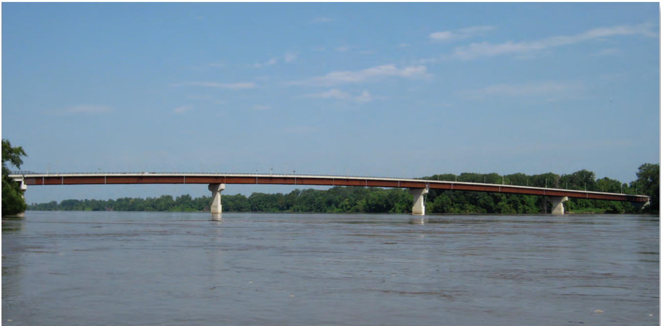
Structure A6288 on State Highway 19 at Hermann, Missouri. Photograph by Joseph Richards, USGS.
