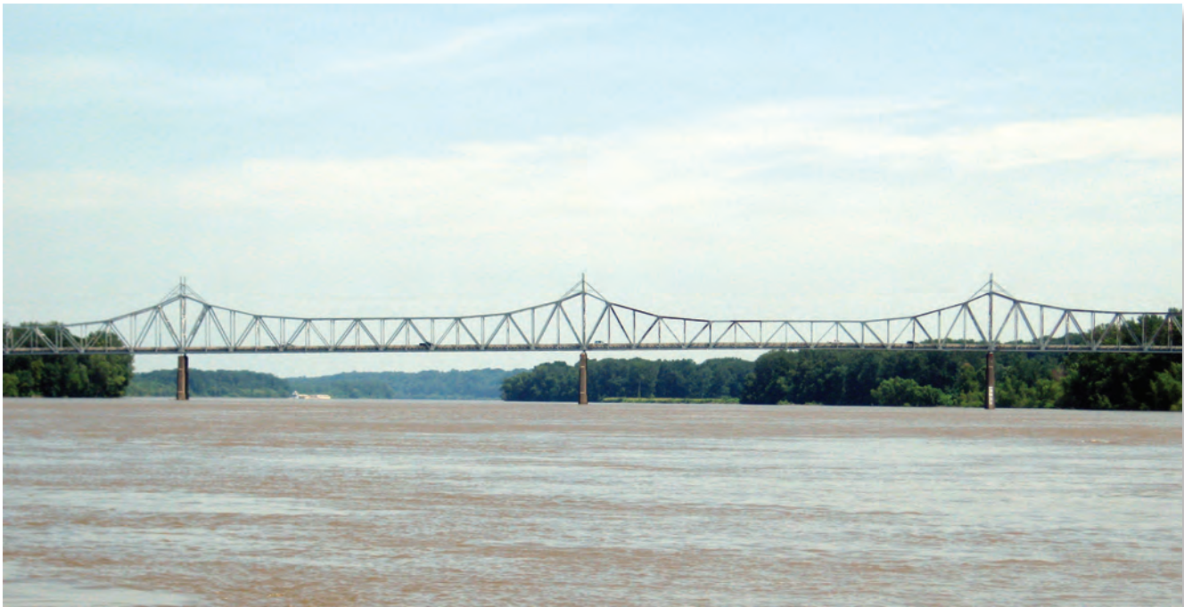
Structure K0969 on State Highway 47 at Washington, Missouri. Photograph by Joseph Richards, USGS.
