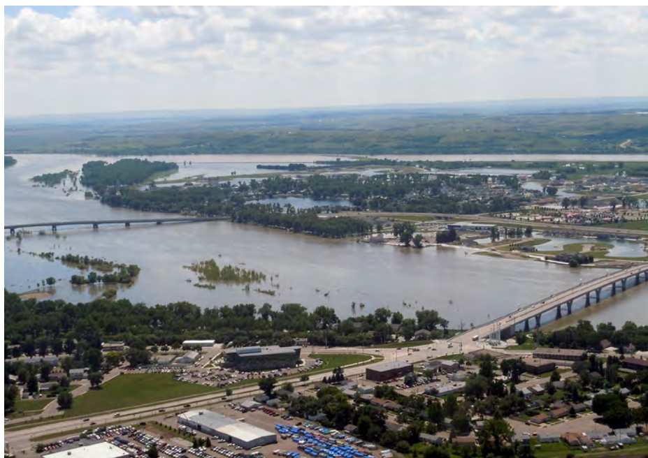
Missouri River at Bismarck, North Dakota (site 2), June 23, 2011. Samples were collected from bridge on right side of photograph (photograph by Joel M. Galloway, U.S. Geological Survey).
