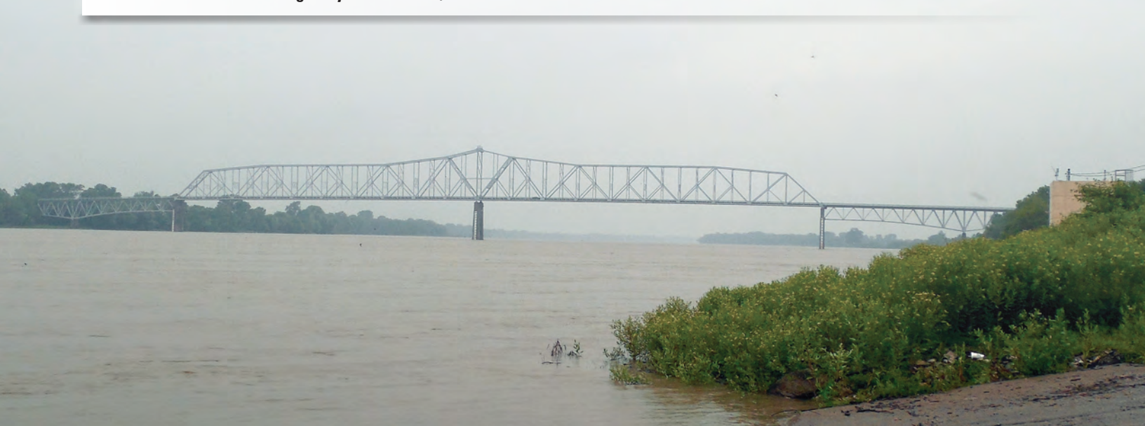
Structure L0135 on State Highway 51 at Chester, Illinois.
