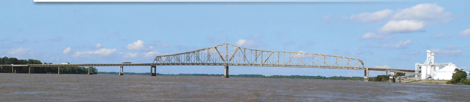
Structure A1700 on Interstate 155 near Caruthersville, Missouri.
