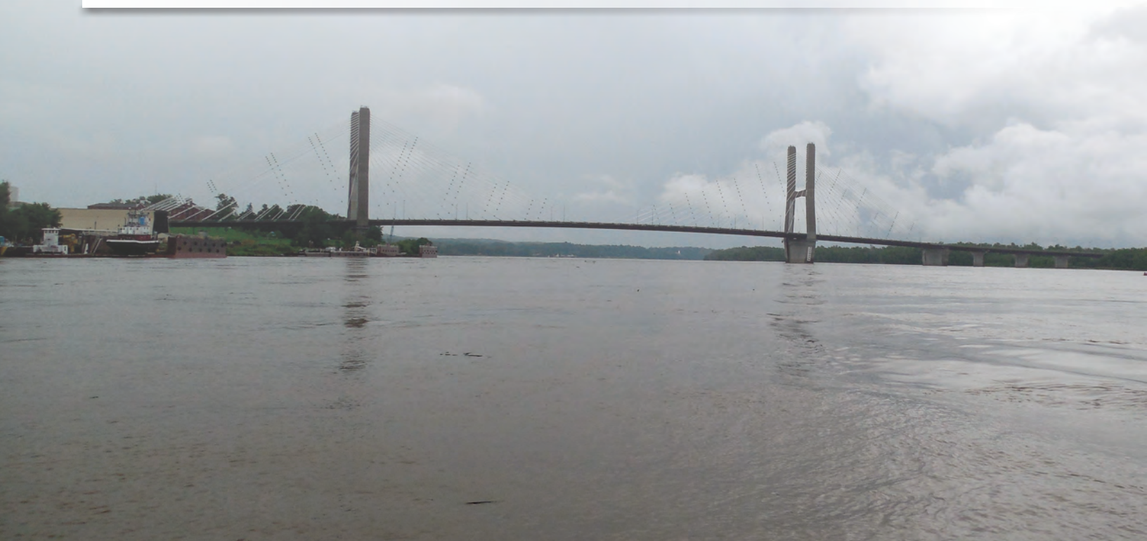
Structure A5076 on State Highway 34 at Cape Girardeau, Missouri.
