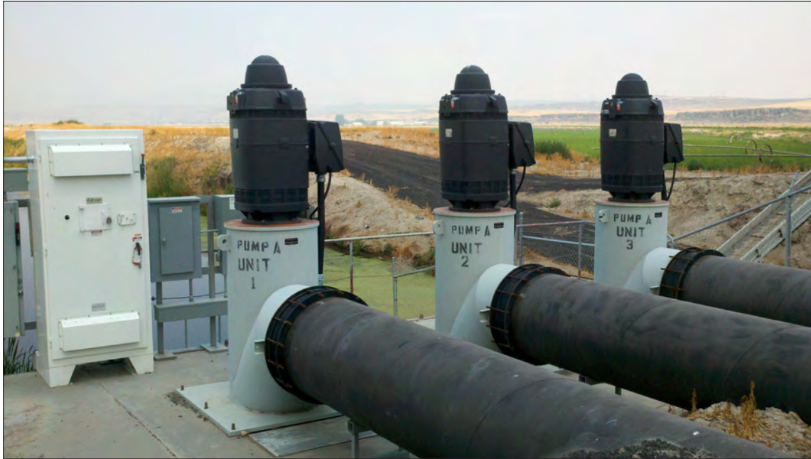
Figure 5. Example of a drain pump (pump A) in the Tulelake Irrigation District system, California. Photograph taken by Esther Pischel, U.S. Geological Survey, July 31, 2013.
