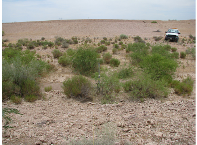
Figure 18. Cross section 2 in the Centennial Wash at Southern Pacific Railroad Bridge near Arlington, Arizona, July 1, 2009.
