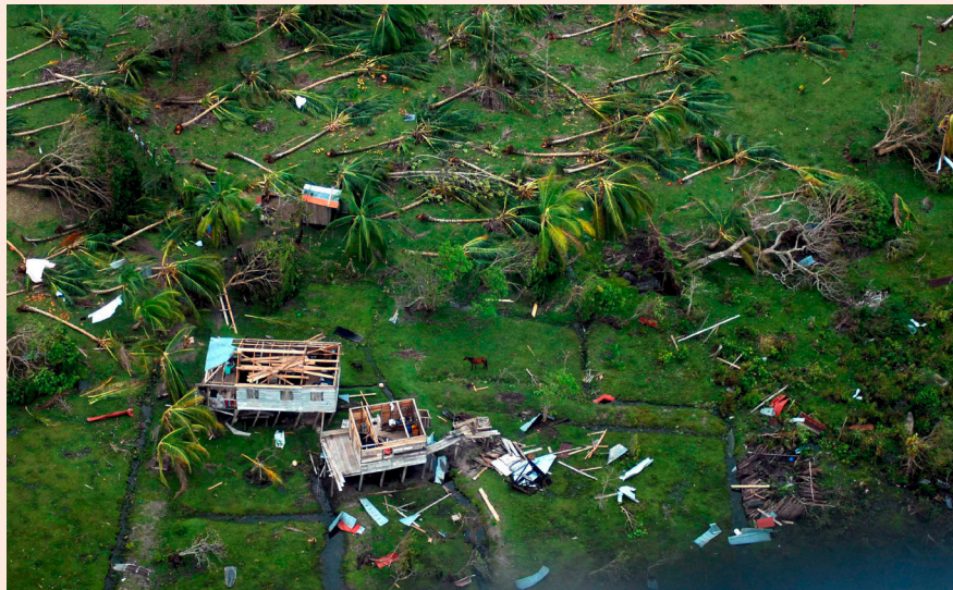
Figure 15: Hurricane Felix destroyed thousands of homes in Nicaragua's low-lying Caribbean coast, leaving dozens dead and dozens more missing. Source: Swiss Re.
