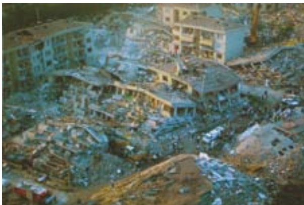
A row of collapsed buildings in Golcuk, Turkey, after the 1999 earthquake. © courtesy of United Nations
