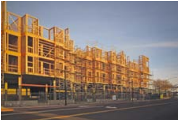
Construction in 2014 of a large four-storey apartment building near San Francisco, California, with three stories in timber construction atop a one-storey RC parking garage. © Randolph Langenbach
