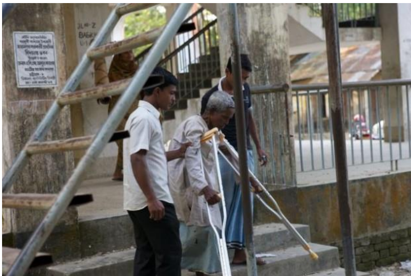
Figure 9: Disaster Risk Management Project (DRM). An elderly person with a disability goes down the stairs of the Cyclone shelter in Mohanagar, Sitakunda, Bangladesh. Photo: IPSnews
