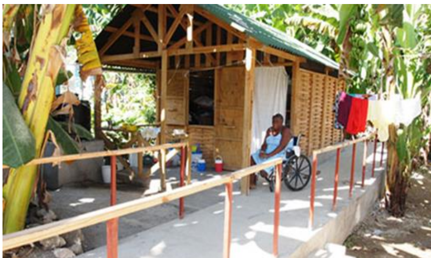
Figure 47: Accessible new housing, along accessible route. Photo: CBM.
