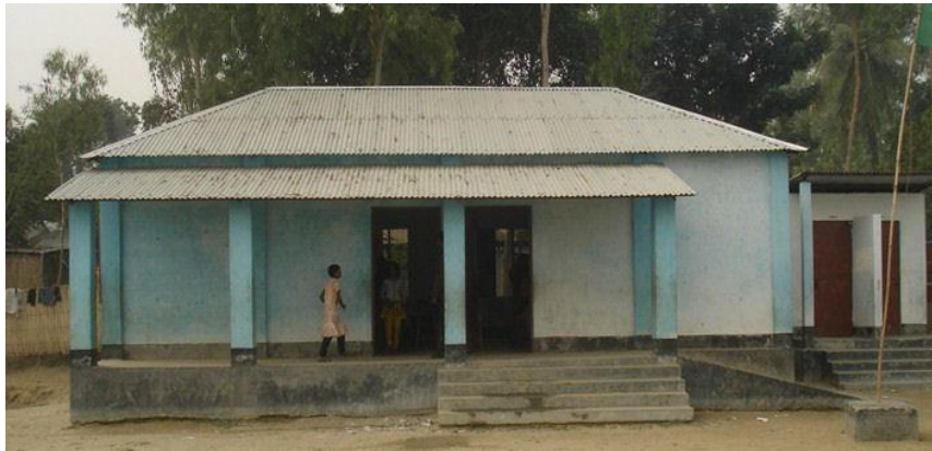
Figure 35: Flood shelter with wheelchair ramp on raised land in Bangladesh. The shelter doubles as a school. Photo: James Pender
