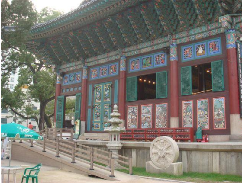
Figure 36 Shrine with accessible ramp. Photo: Betty Dion
