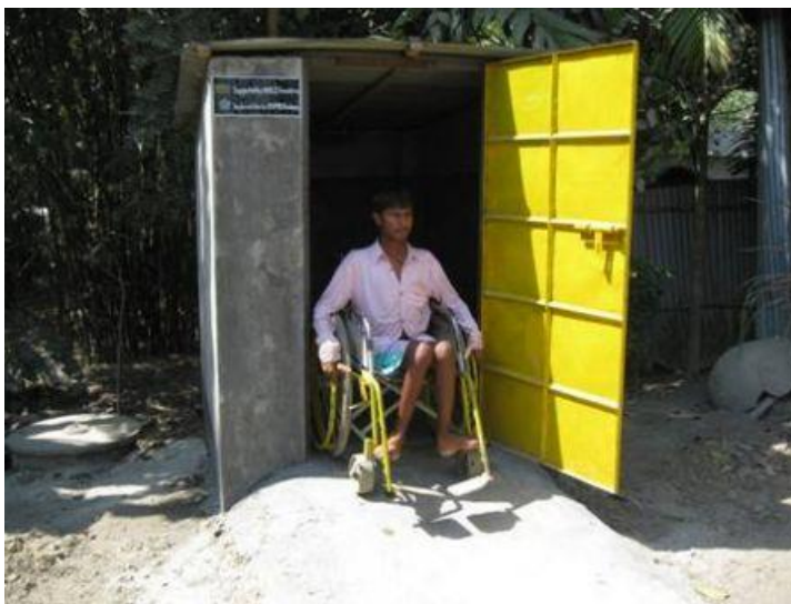
Figure 78: New sanitary facility with ramp and door opening outwards. Photo: Abilis
