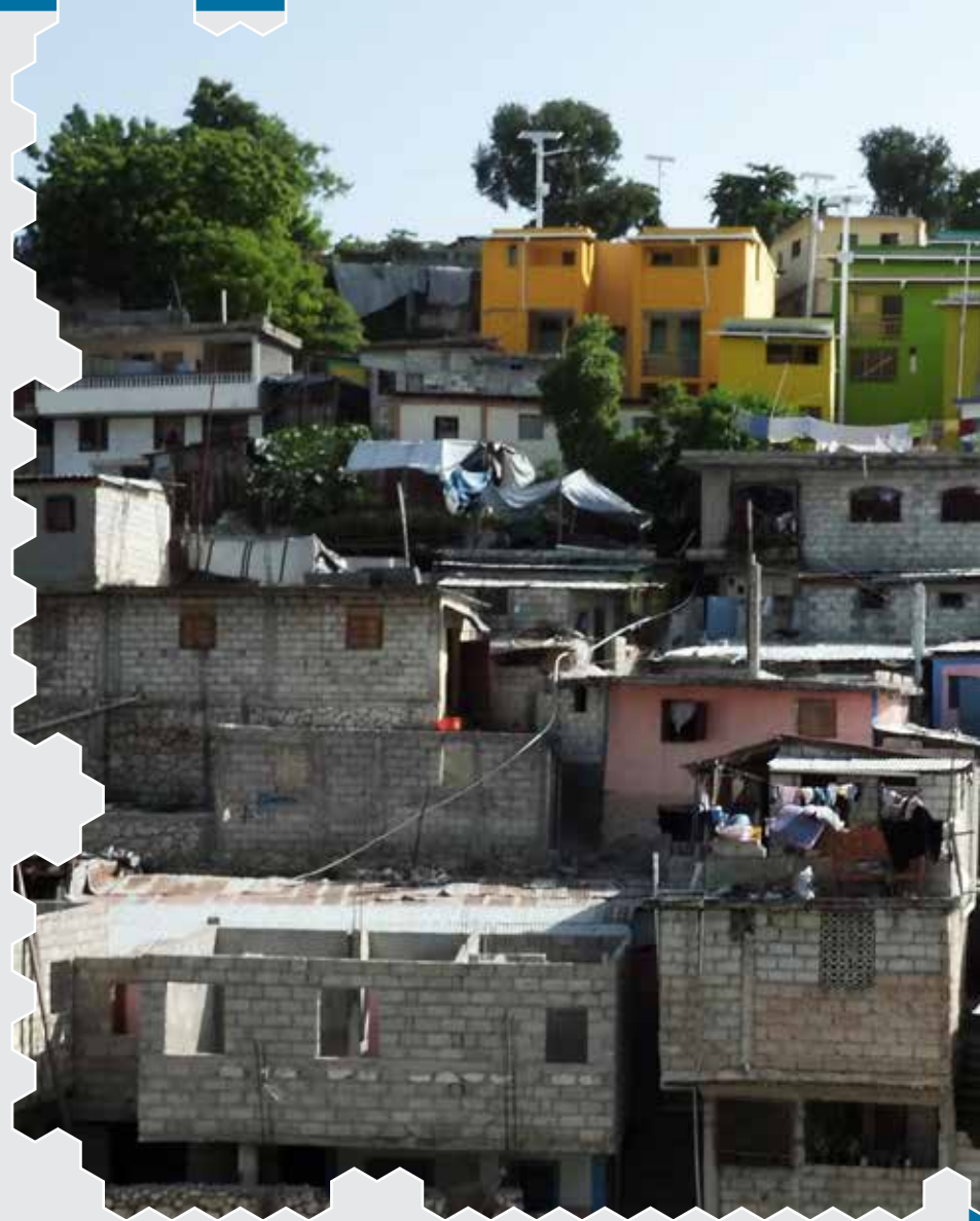
Photo : One of the objectives of the collaboration between the Haitian government and the United Nations in the 16/6 project was to rebuild targeted earthquake affected neighbourhoods so that they could withstand further tremors, making it easier for the people who had been displaced by the earthquake of 12 January 2010 to return.
